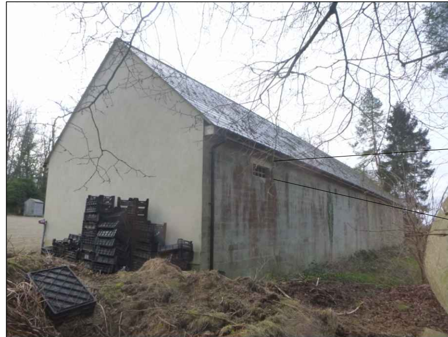
Photograph 2: Showing the western (rear) and northern (gable) elevations for the barn.
