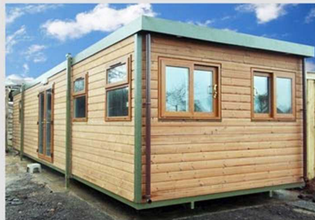
Thermowood timber external cladding
