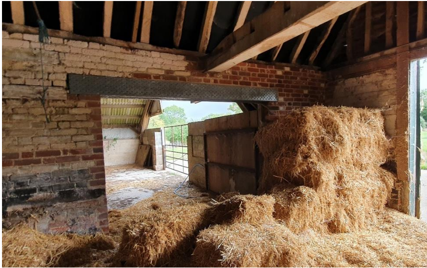
Figure 21 – New opening through existing wall
