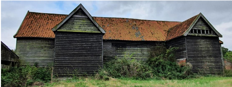
Figure 40 – rear elevation of Barn 3
