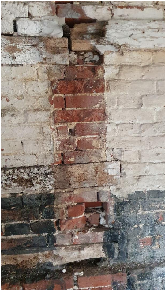
Figure 18 – Bond timber and pier removal
