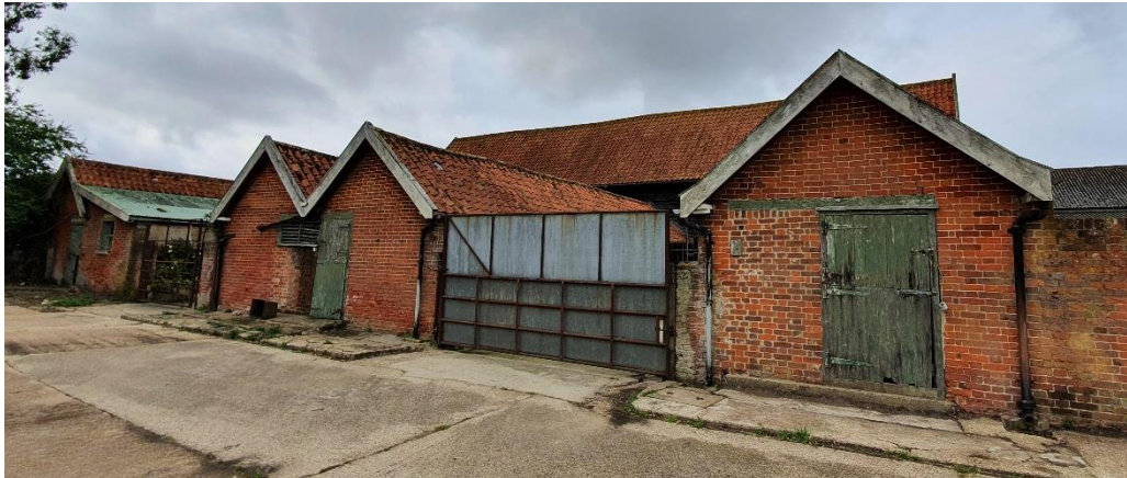
Figure 26 – Barn 3 outbuildings along front elevation
