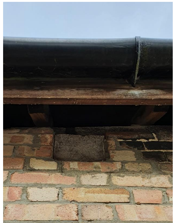
Figure 25 – Eaves & exposed timber beam end
