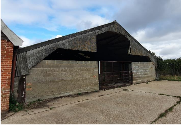
Figure 2 – Barn 1 front view
