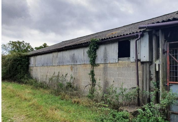
Figure 3 – Barn 1 rear view
