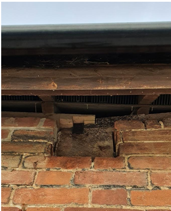
Figure 24 – Eaves & exposed timber beam end
