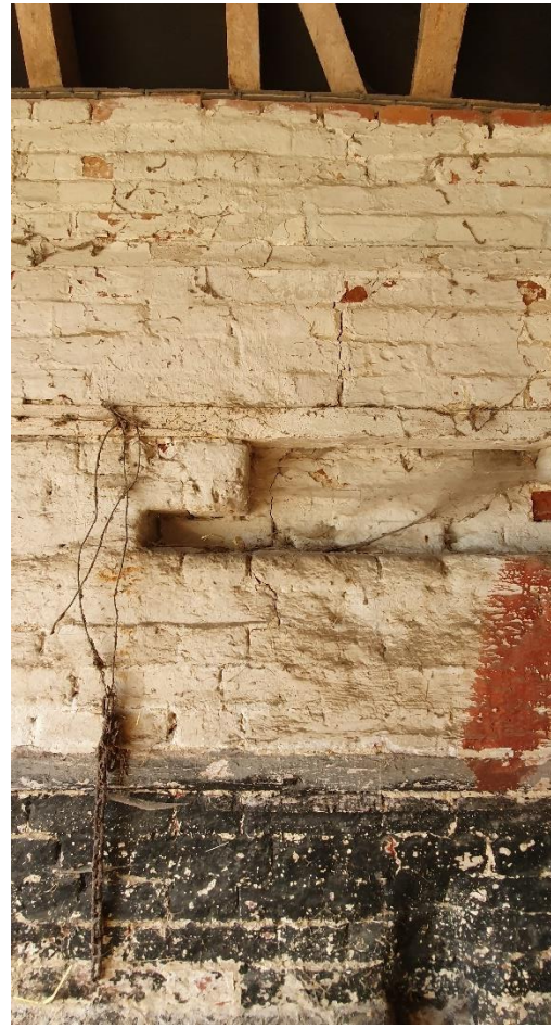
Figure 19 – Bond timbers and voids in masonry
