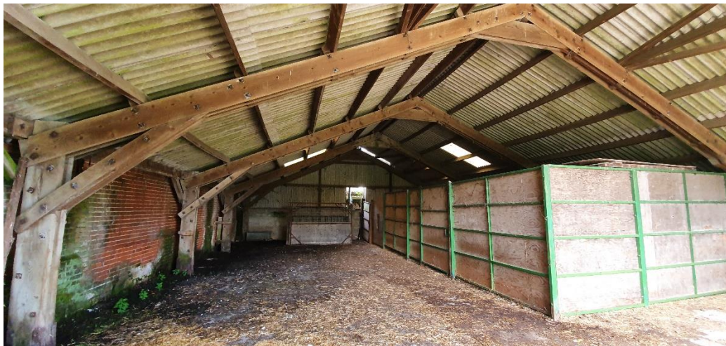
Figure 4 – Barn 1 internal view
