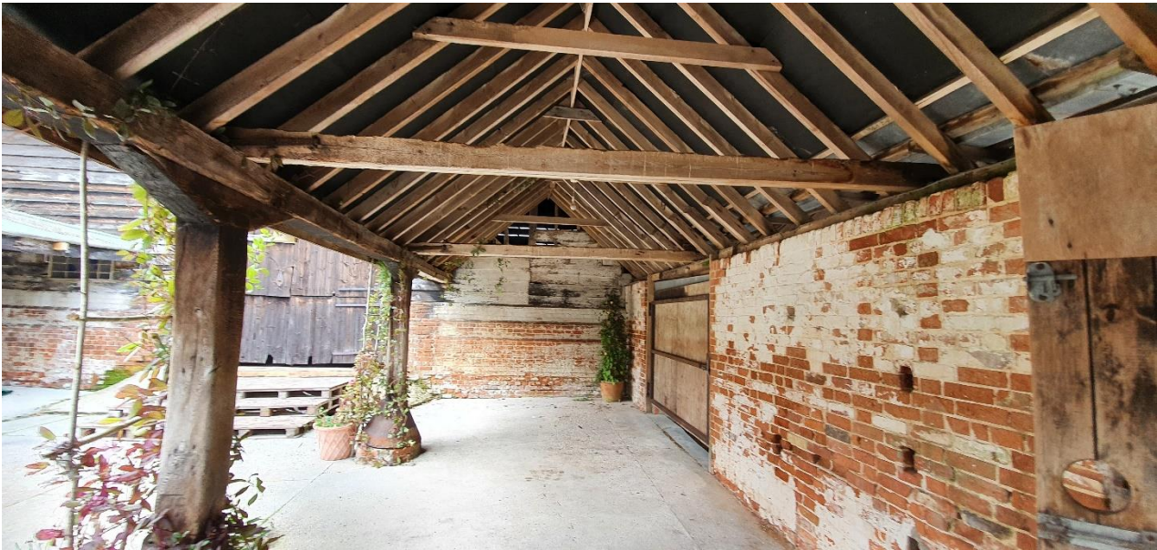
Figure 32 – Outbuildings in courtyard area
