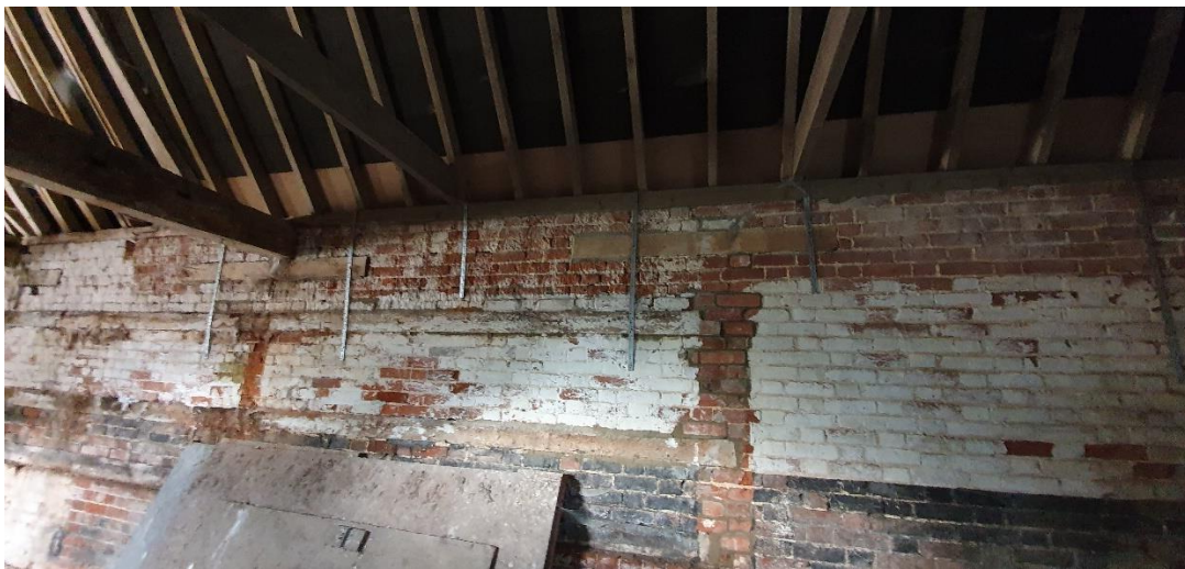
Figure 17 - Replaced roof structure
