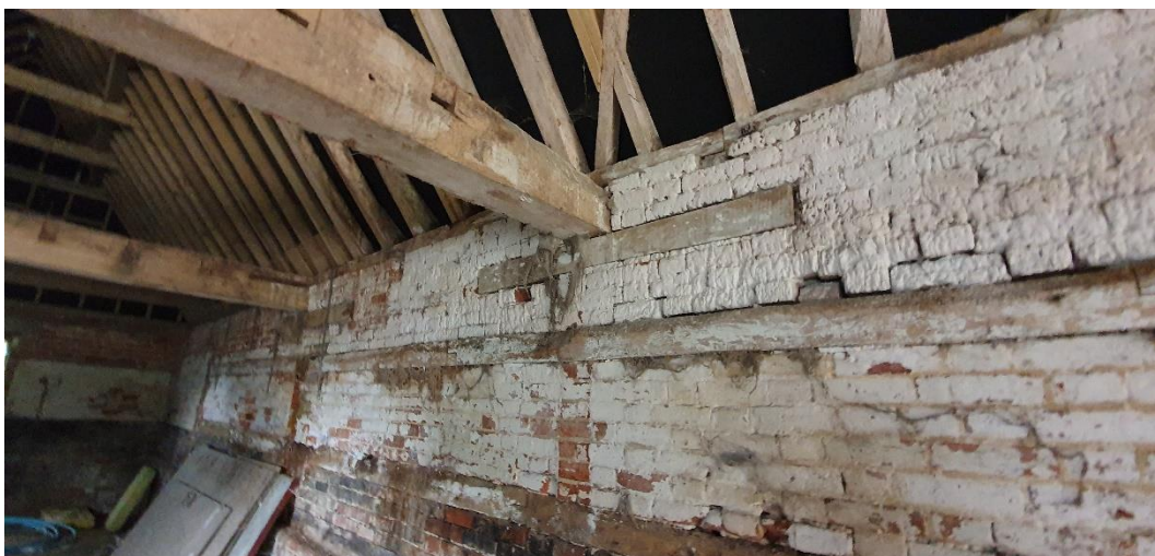
Figure 20 – Bond timbers and timber spreader beams
