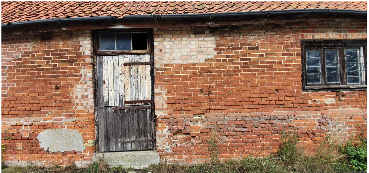
Figure 23 – Barn side view
