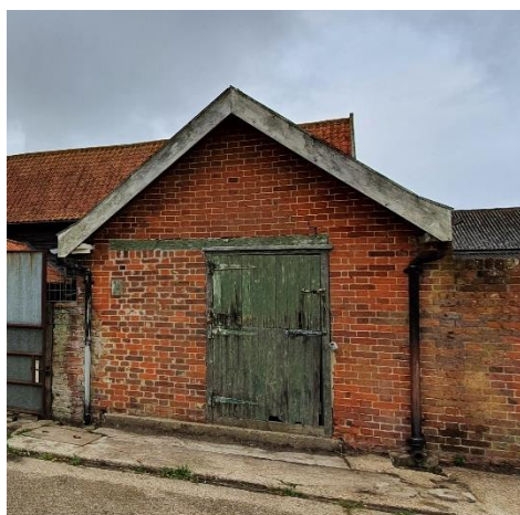
Figure 28 – Outbuilding front elevation
