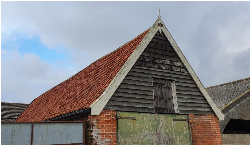
Figure 22 – Clay pantile roof
