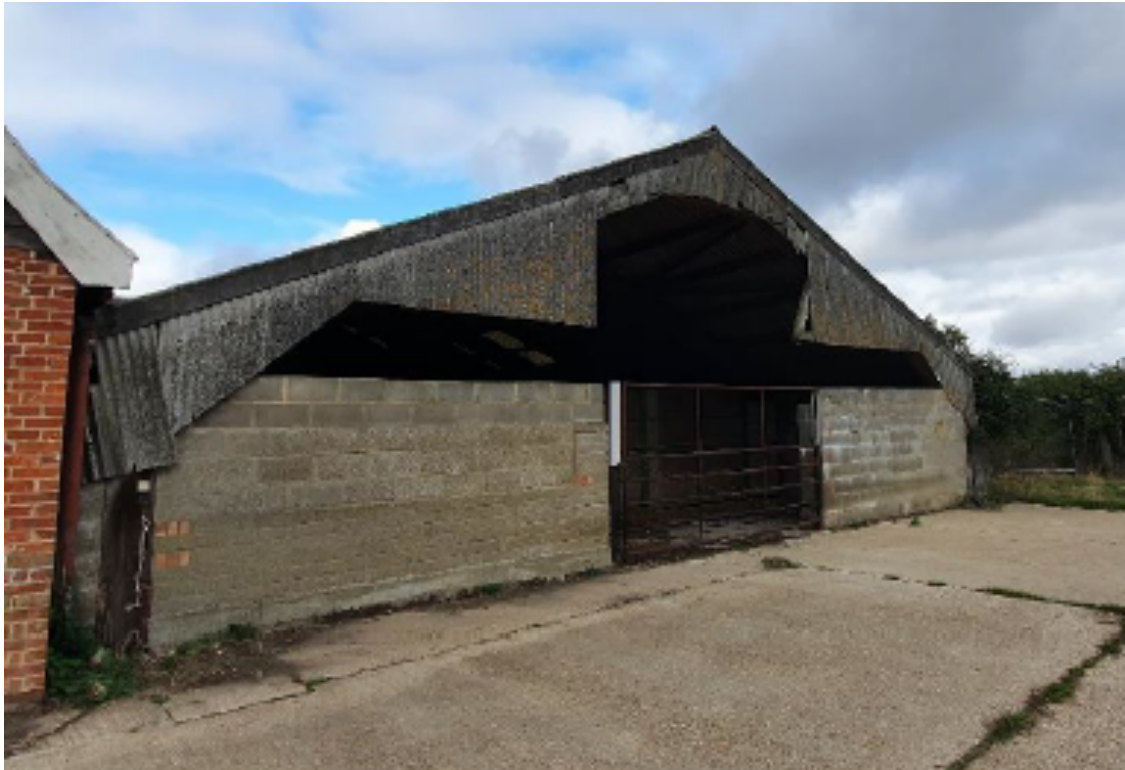
Picture 3 – Front elevation of the barn to be converted to a dwelling
