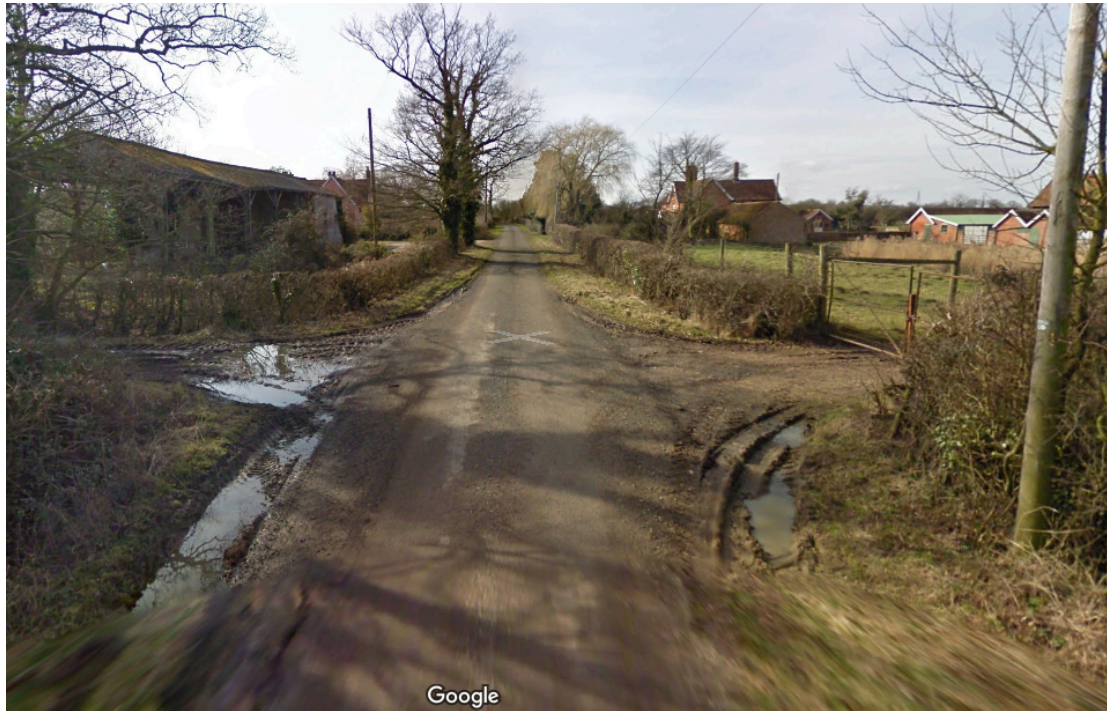
Picture 7 – The existing vehicular access (right) onto Otley Road that will be used by the new dwelling, looking west.
