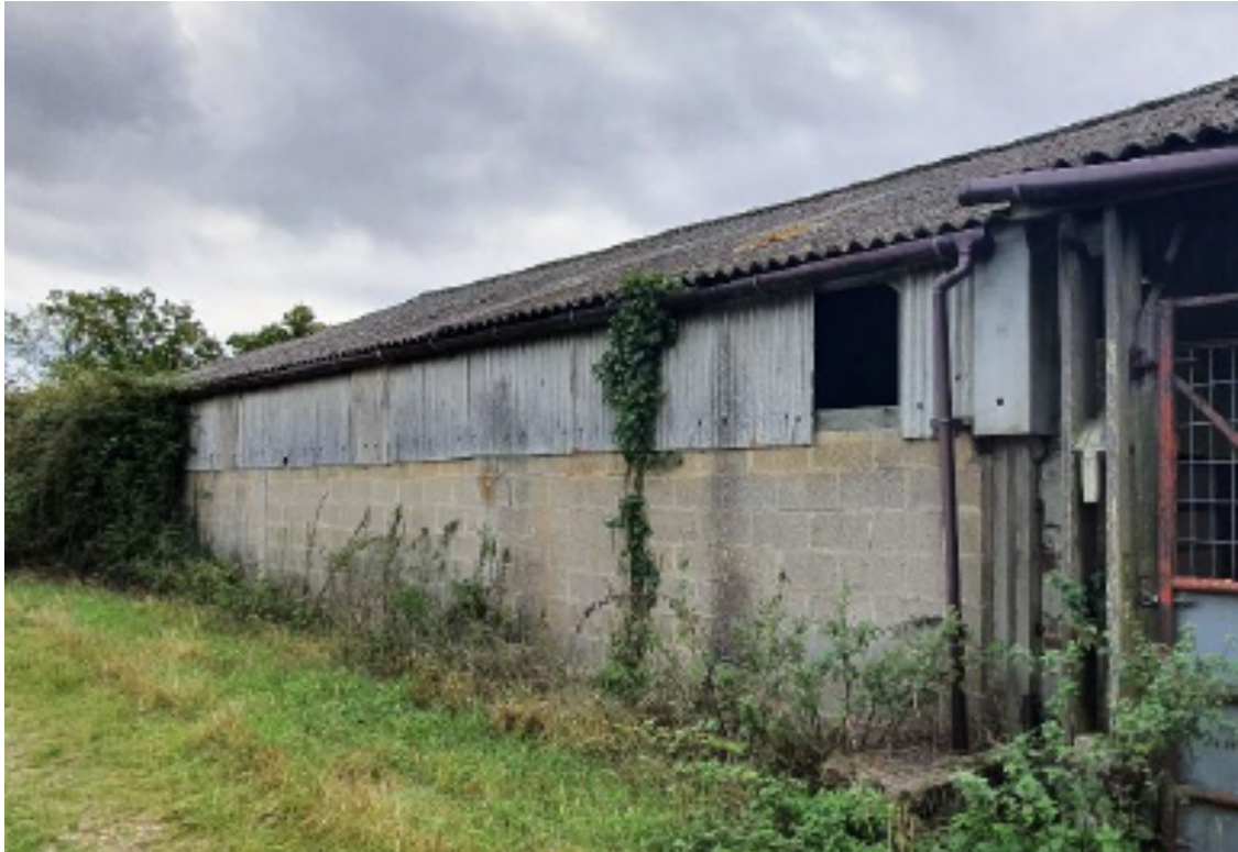
Picture 4 – Rear elevation of the barn
