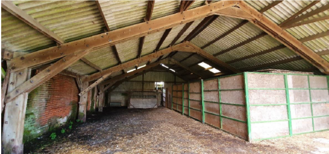
Picture 5 – Internal view of the barn
