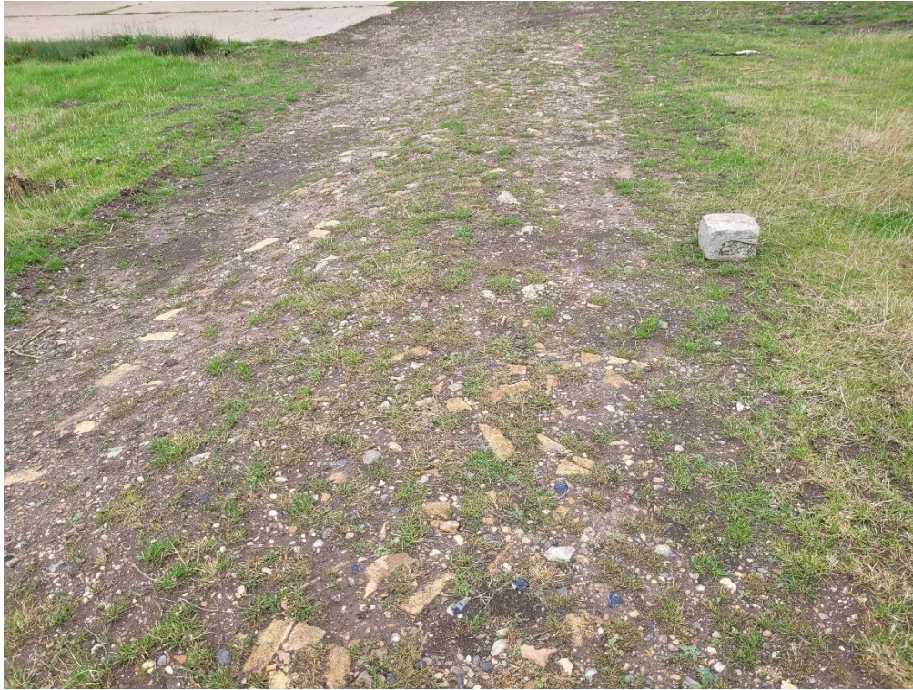
Photograph 7 – Hardstanding track at entrance to site.
