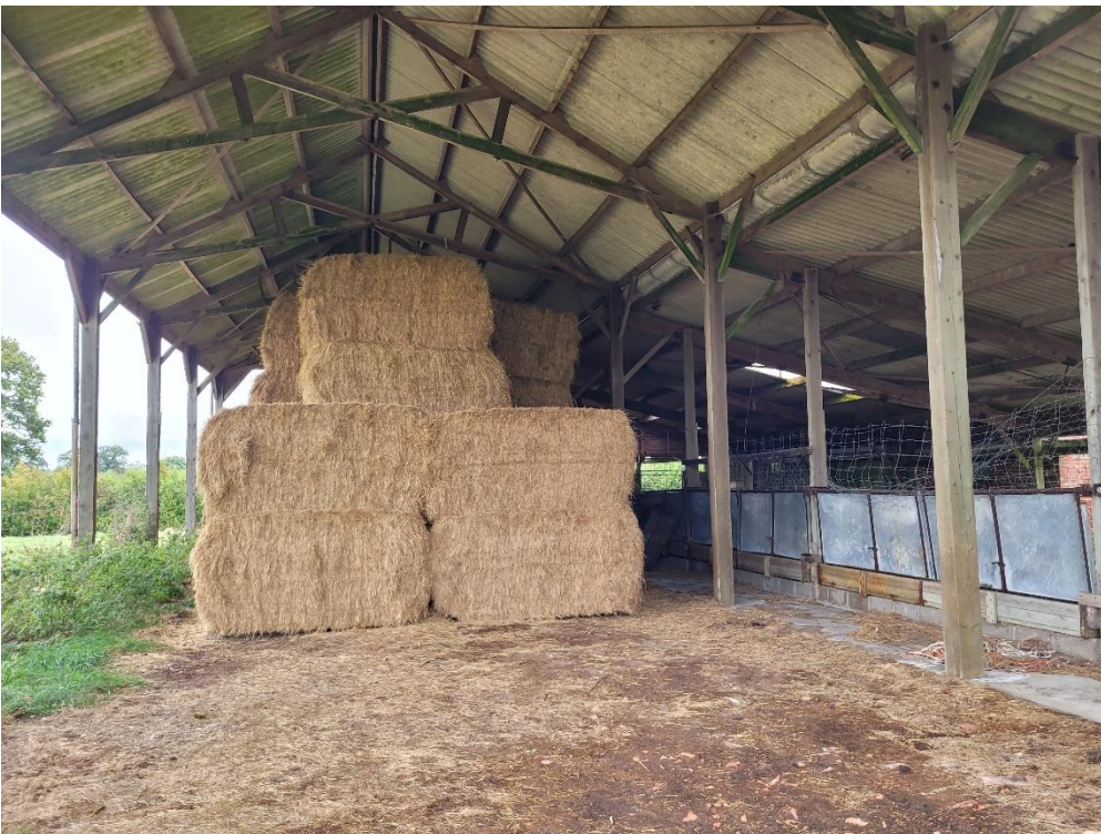
Photograph 4 – Part of Building 8 being used for hay storage.
