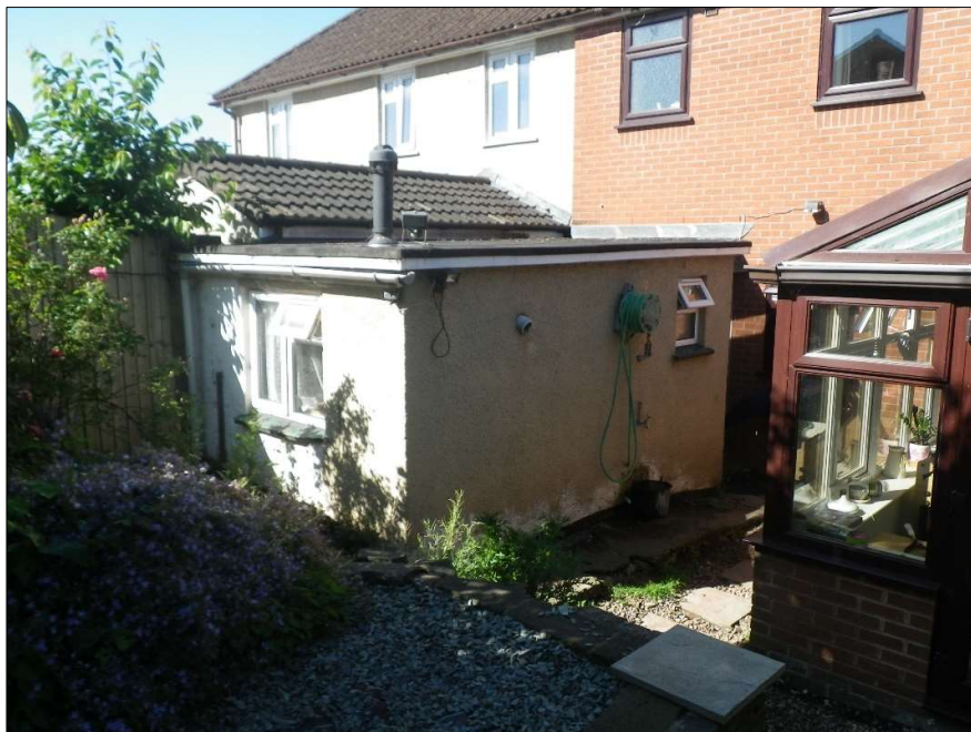
The outhouse: northern and eastern elevations
