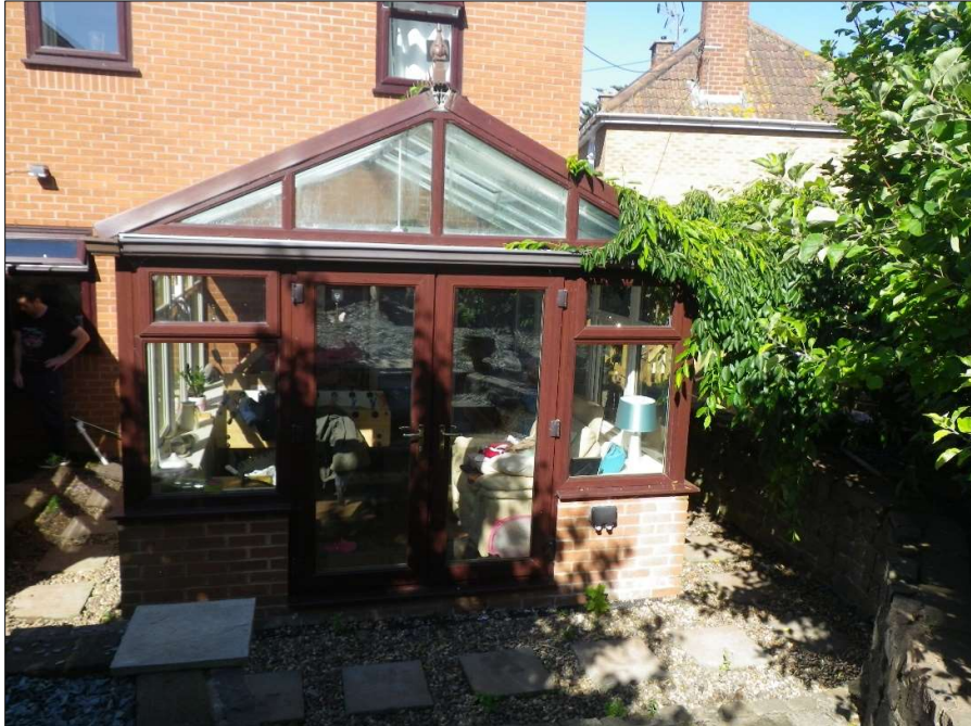
The conservatory: eastern elevation
