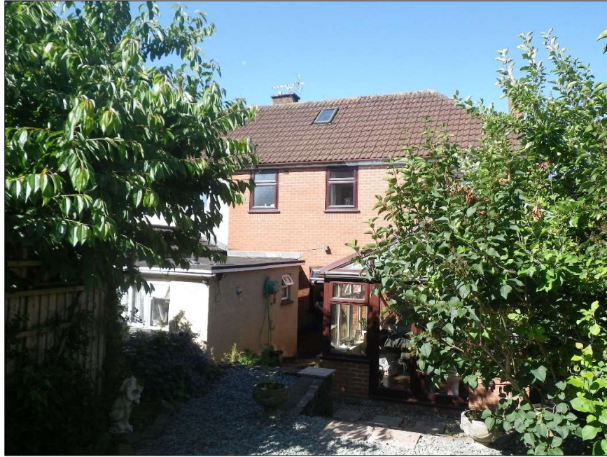
The survey site (eastern elevation)
