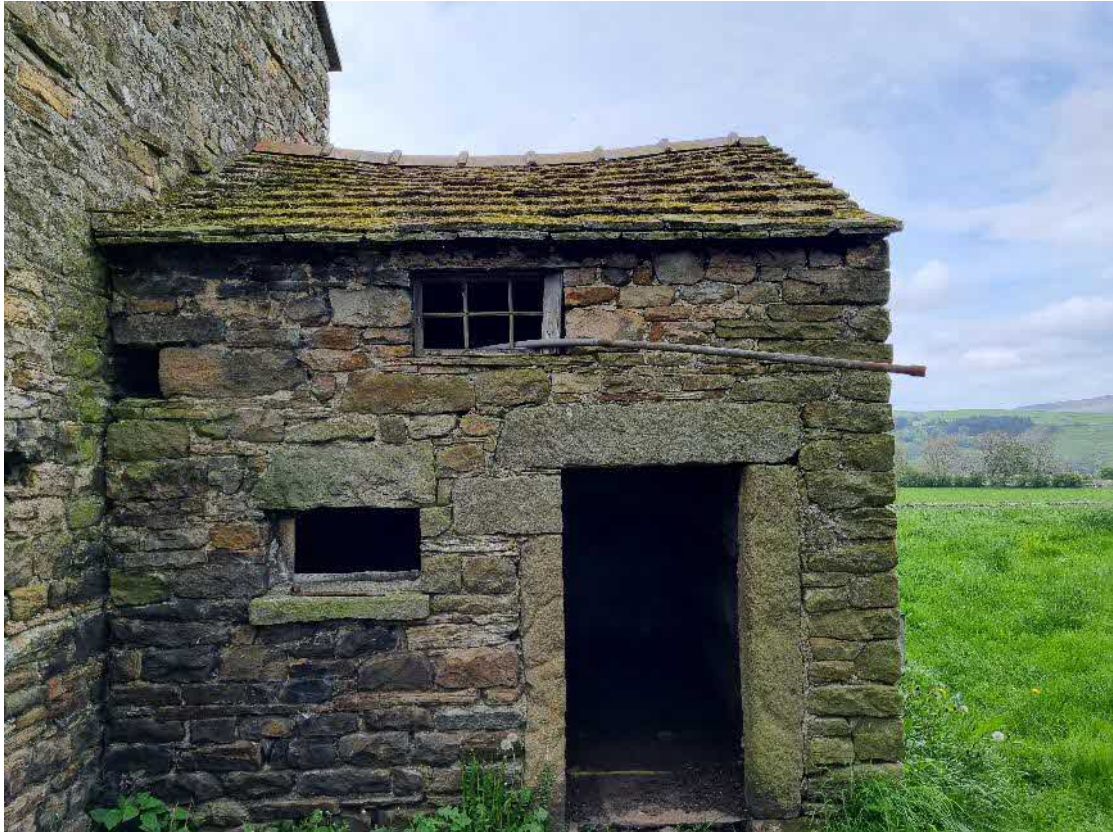
Image 22 – southern elevation of B2 showing PRFs in brickwork and roofing
