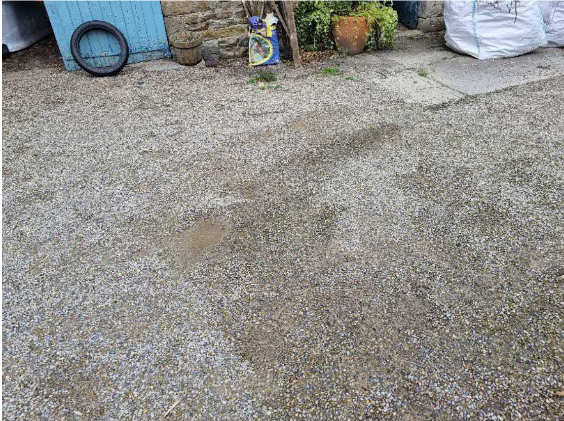
Image 17 – hardstanding driveway to southern aspect of site
