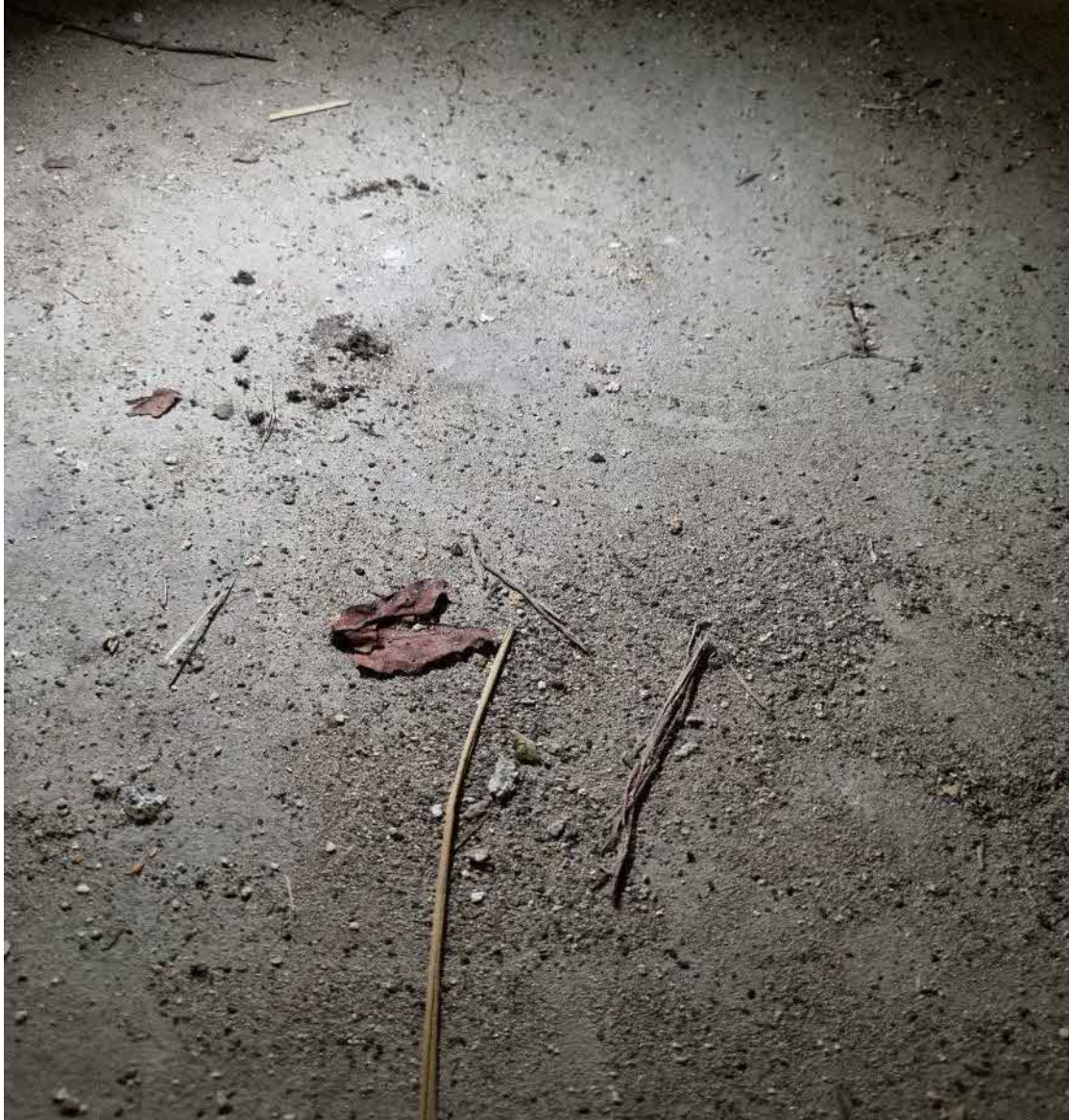
Image 4 – further bat faeces present on floor of eastern end of B1
