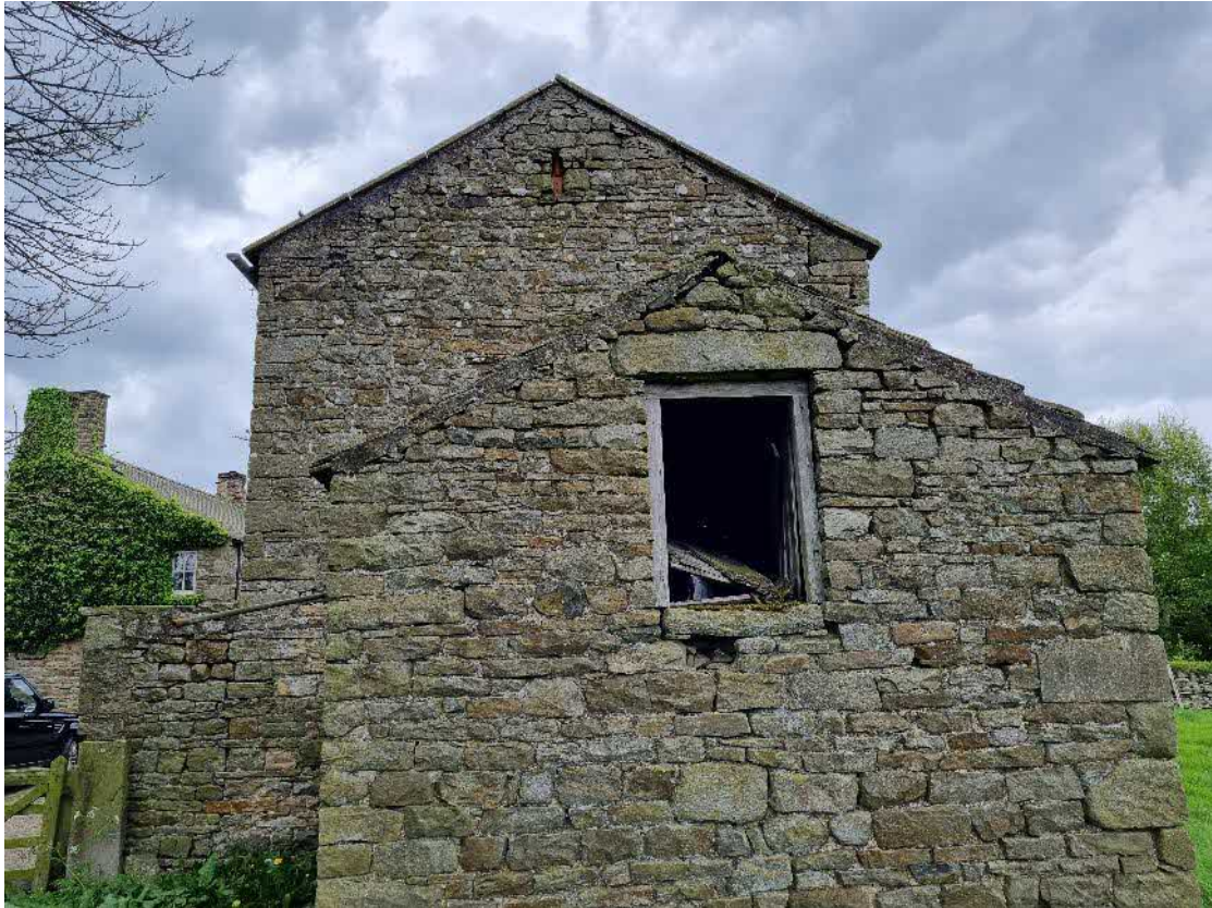
Image 23 – eastern elevations of B1 and B2 showing PRFs in brickwork
