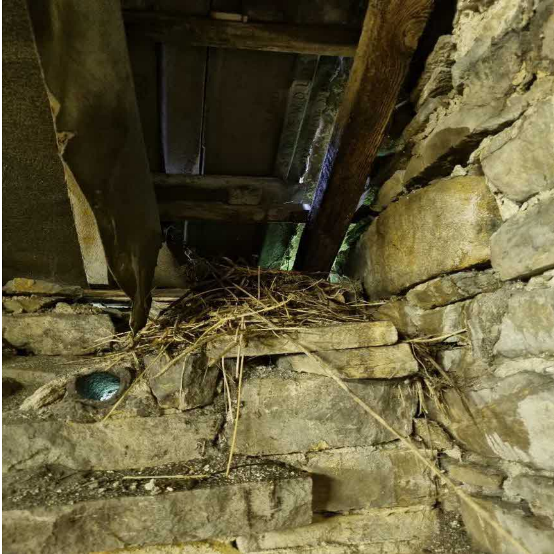
Image 7 – possible jackdaw nest, thought to be inactive at time of survey
