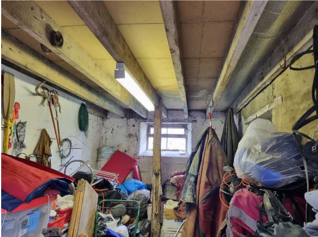
Image 21 – internal space on ground floor of B1 used for storage
