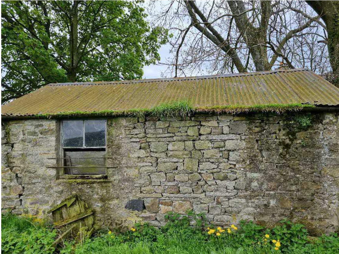
Image 14 – northern elevation of B2 showing PRFs visible in external brickwork
