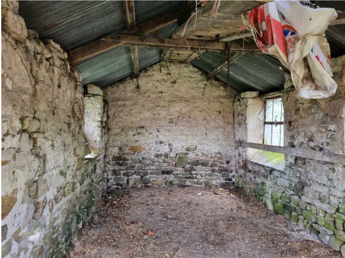
Image 13 – interior of B2 showing some PRFs in brickwork
