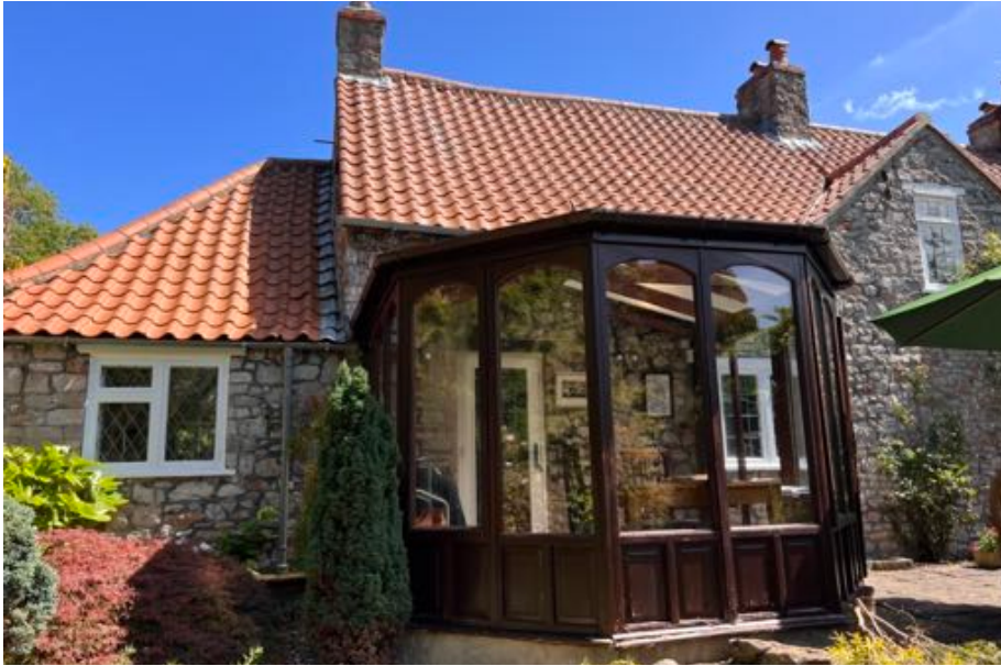
Plate 2. North-western elevation of conservatory for demolition
