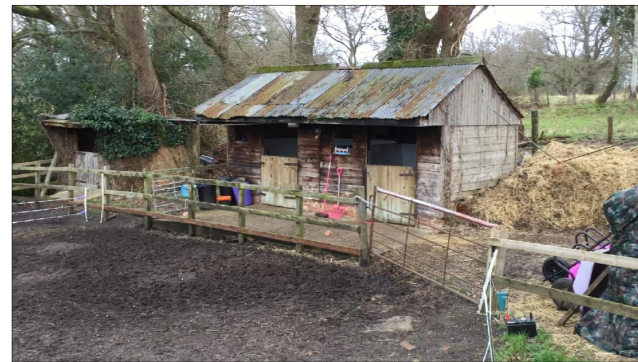
PHOTO OF THE EXISTING STABLES
