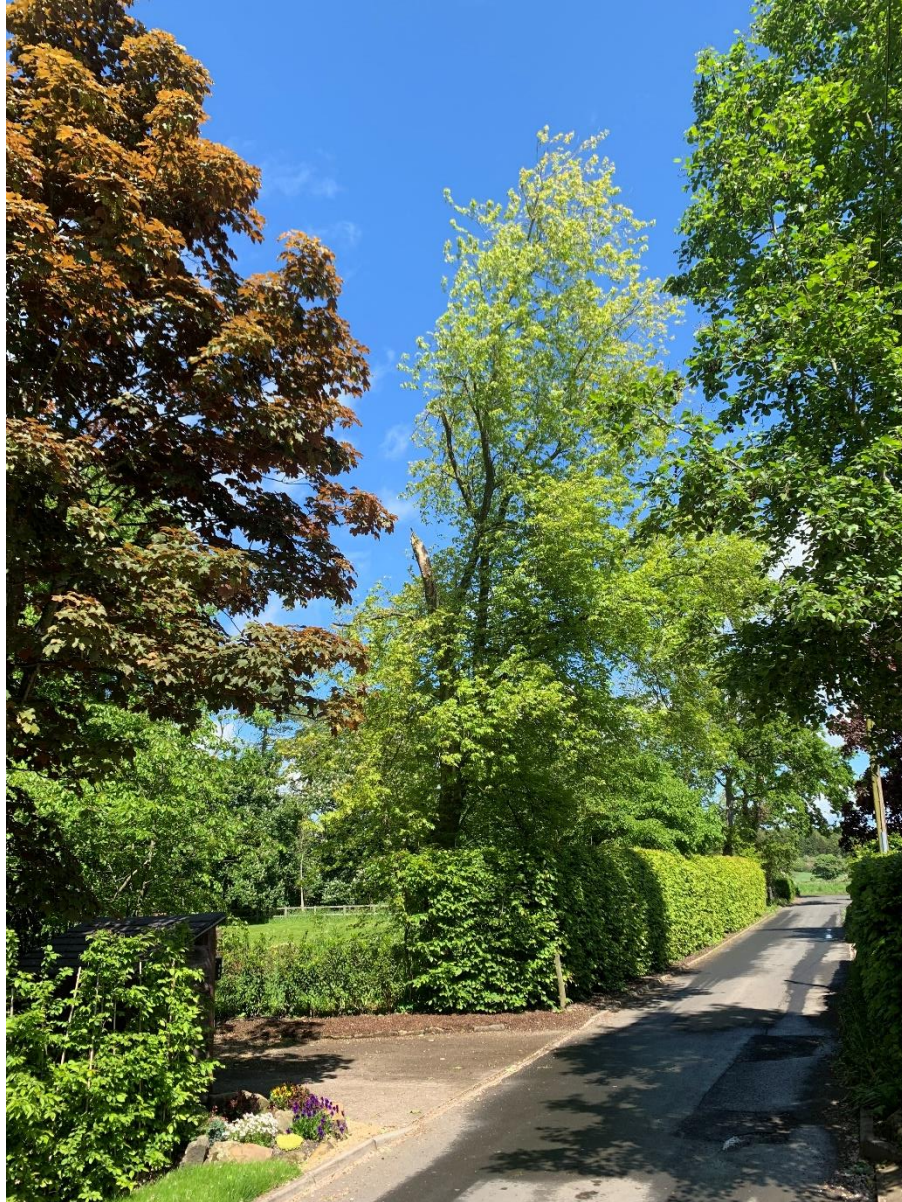
Above: Tree T10, storm, damaged crown.
