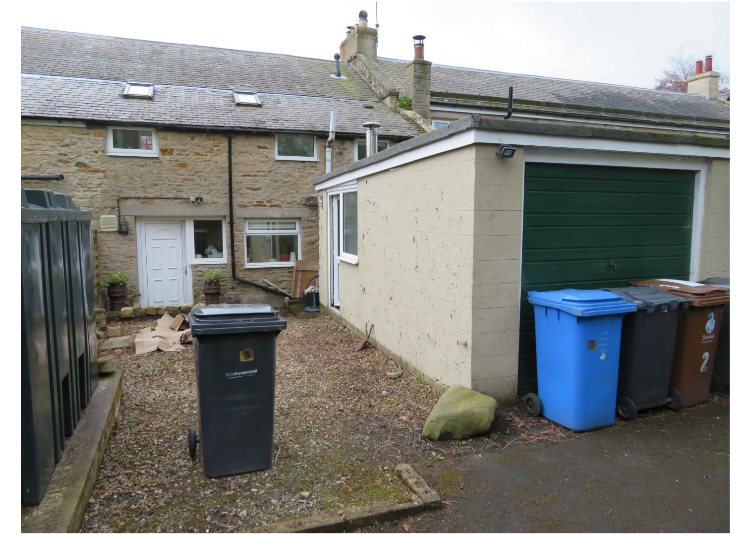
General photo of the rear elevation/garage block
