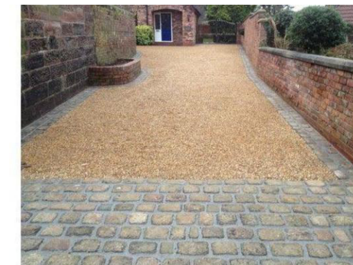
GRANITE SETTS TO GATE ACCESS
