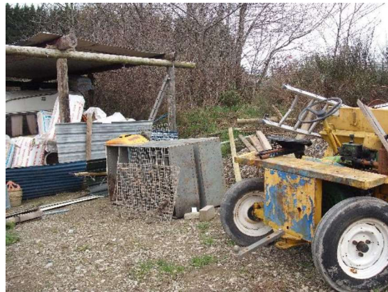
Photo 5: temporary roofed area in front of cutting
