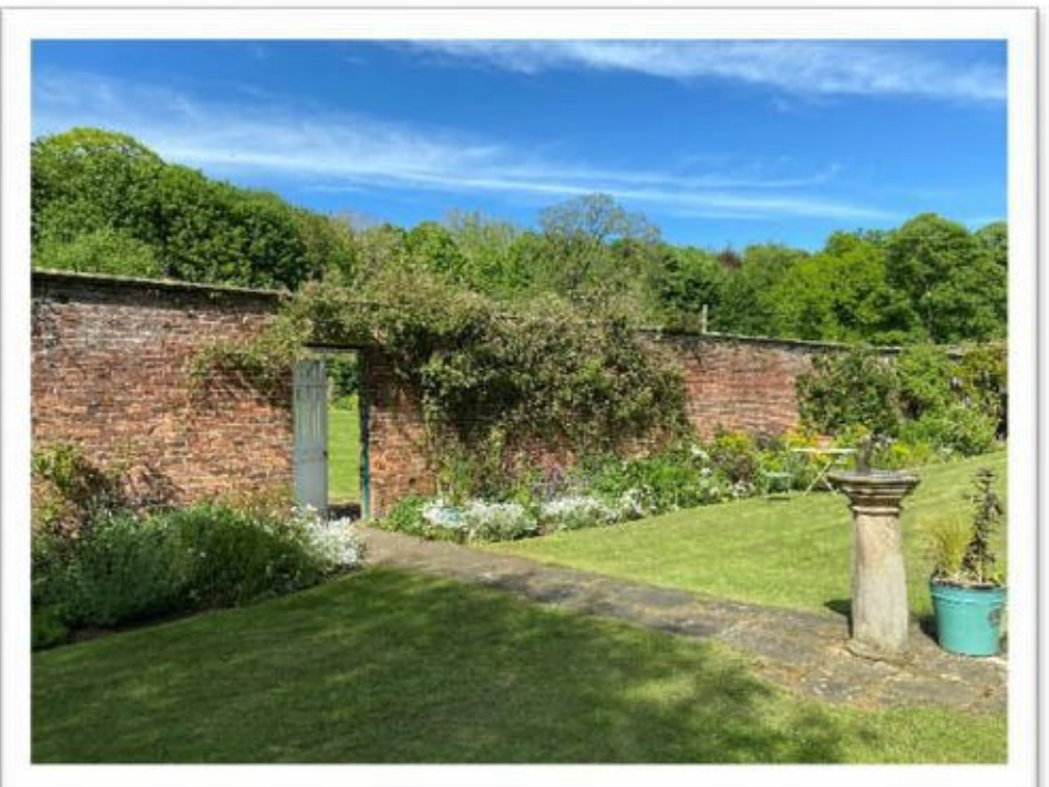
Figure 3 The walled garden south doorway and southern wall
