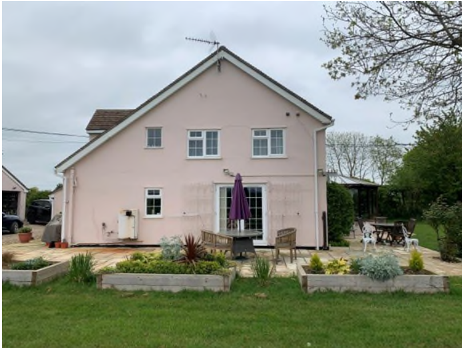
Rear Southwest elevation
