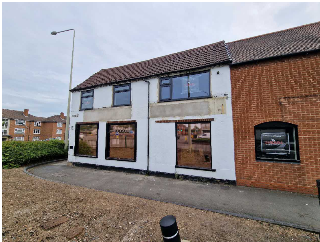
Plate 10: West elevation – detail of windows
