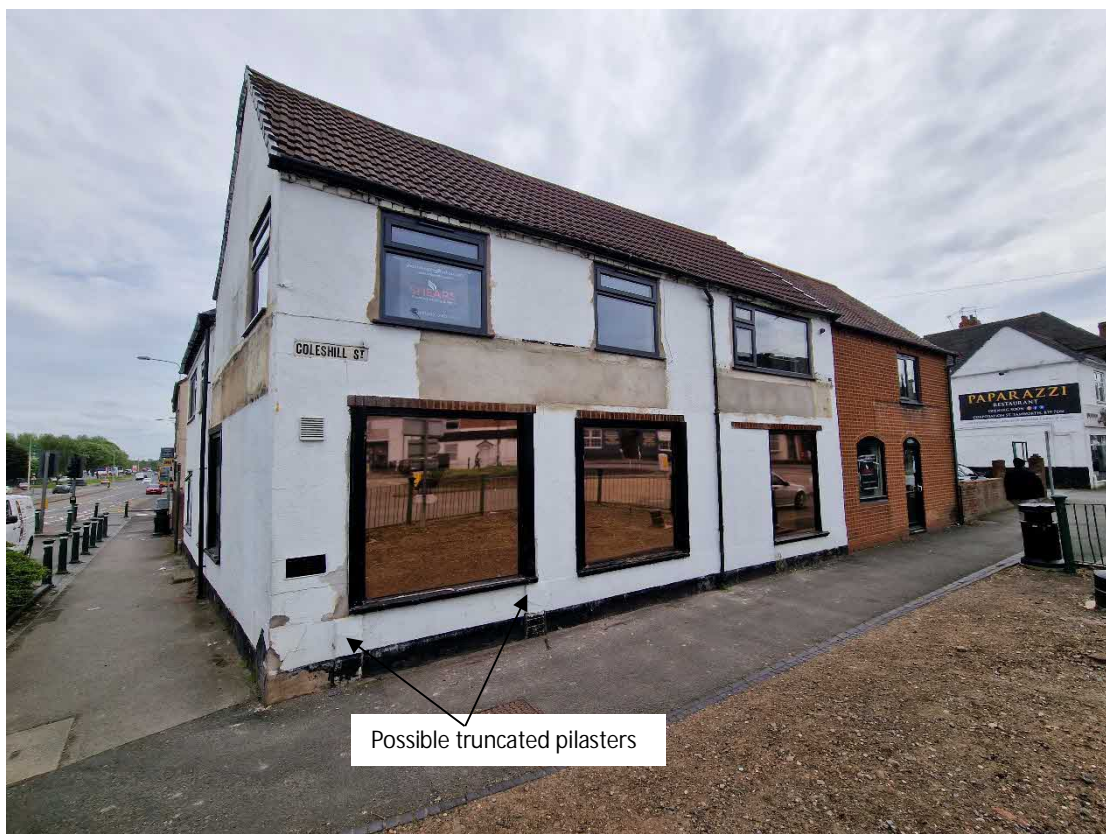
Plate 9: General view of the west elevation
