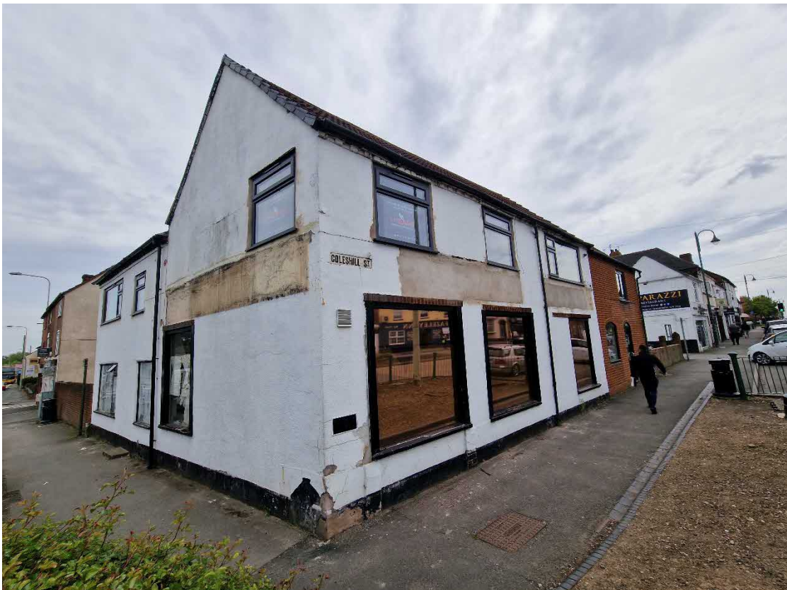
Plate 6: General view of the north and west elevations
