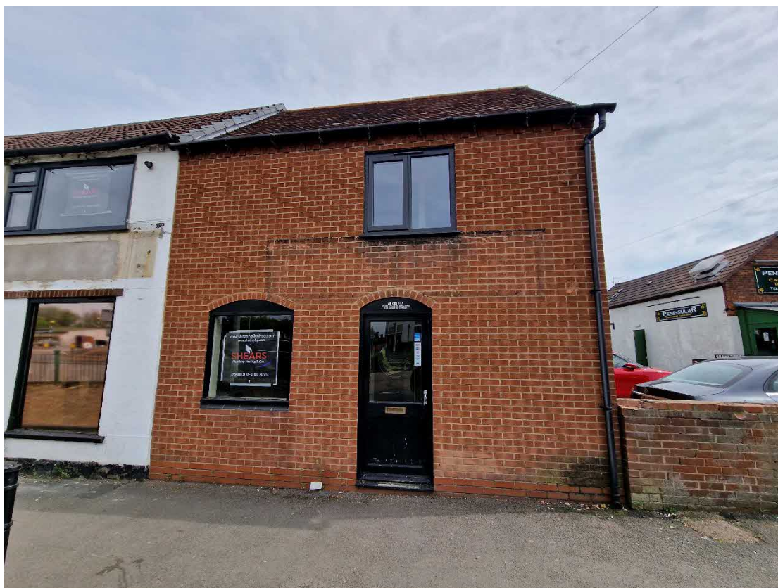
Plate 12: West elevation – detail of later south extension
