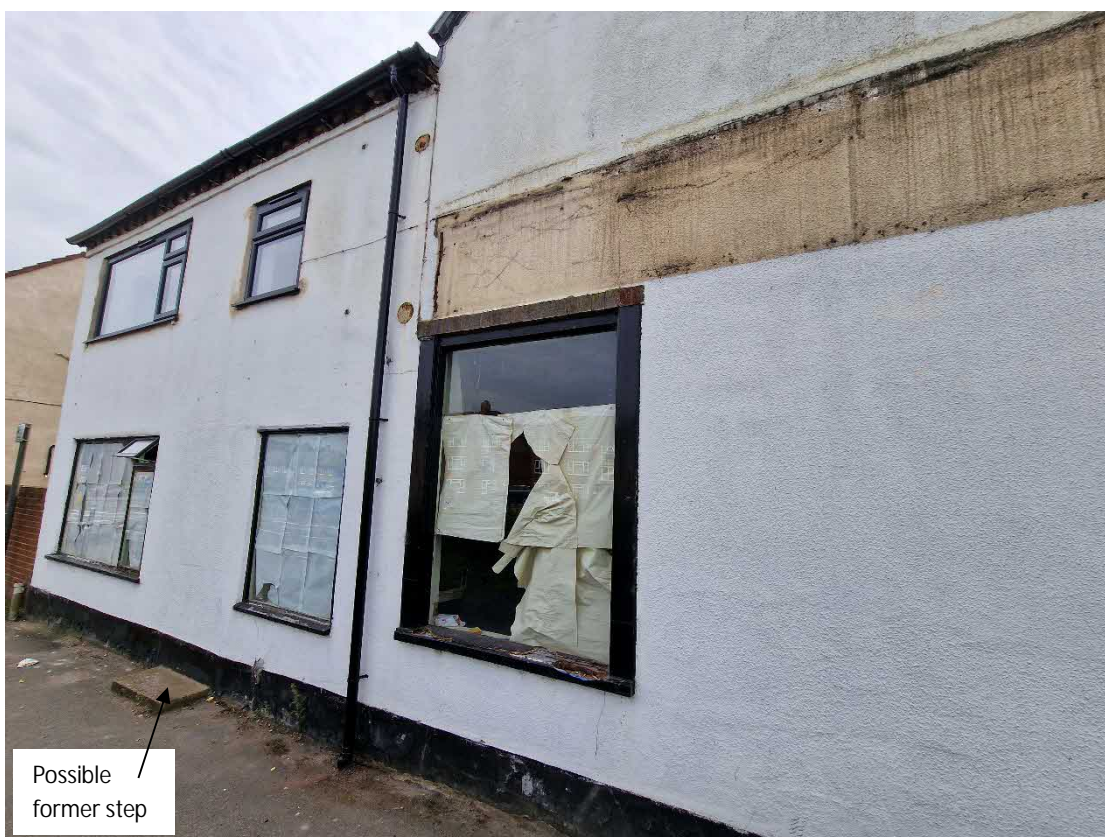
Plate 8: Detail of windows within the north elevation and possible step (arrow)
