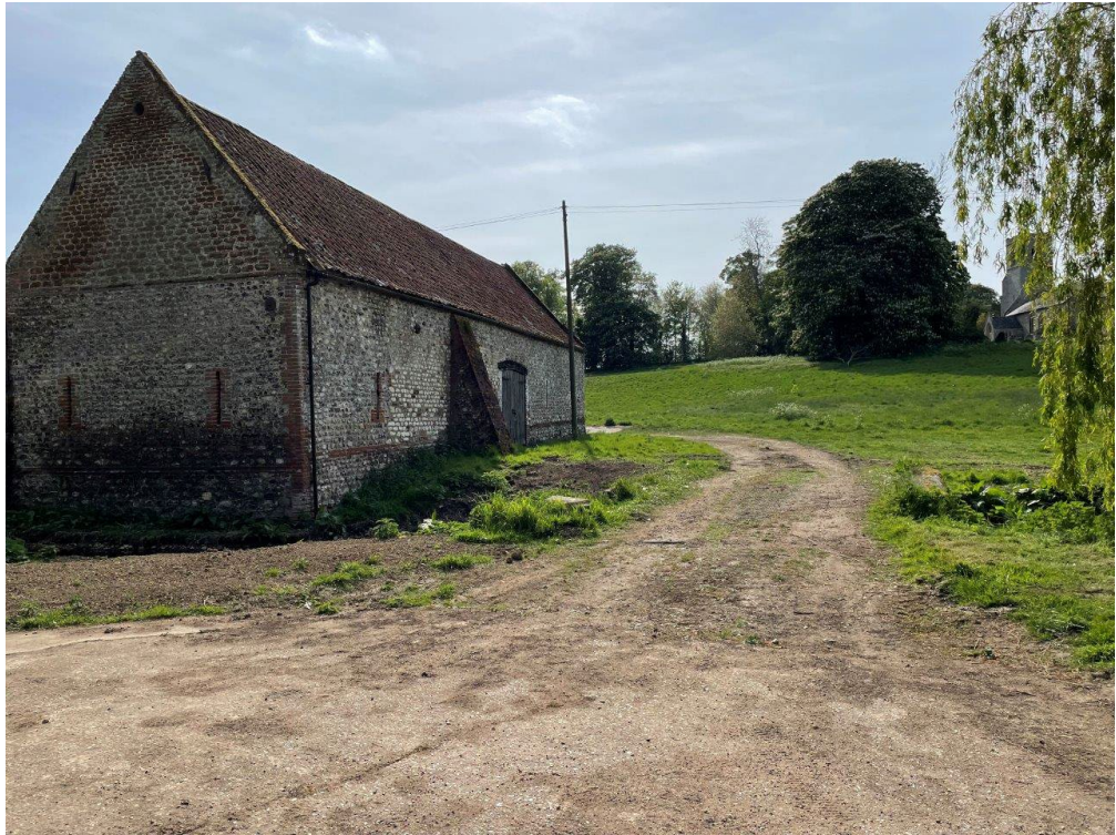
Image 10 (above): East facing gable and northern elevation of field barn
