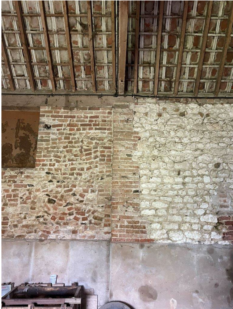
Image 12 (above): Internal view of south facing elevation of Field Barn. Photo shows existing opening in wall, original brick quoin and (to left of quoin on image) irregular brickwork infill where former opening has been infilled, with timber lintel over original opening above.
