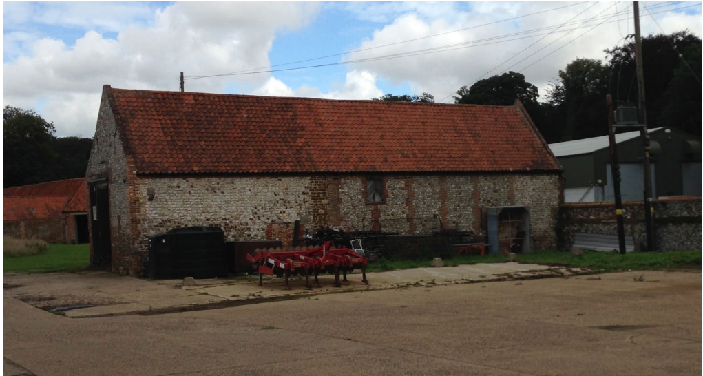
Image 8 (above): Southern elevation of Field Barn
