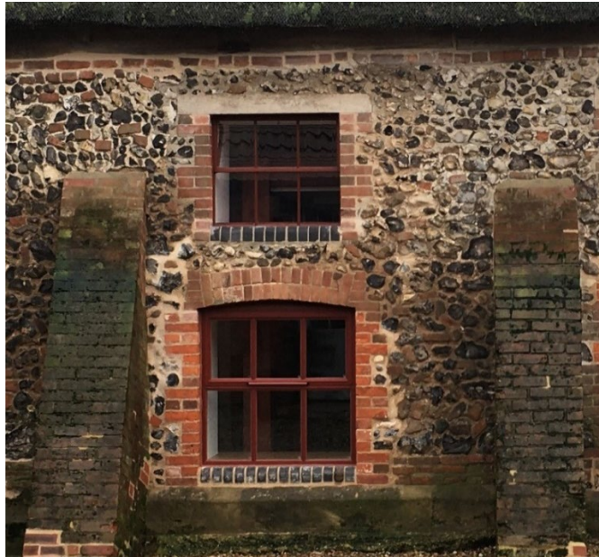
Image 13: Example of 'W20' upper and 'W40' lower window frame
