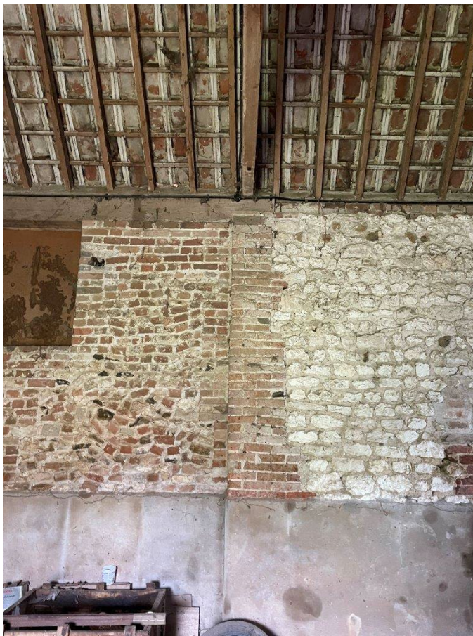
Photo 6 Interior – showing infilled doorway in southern elevation
