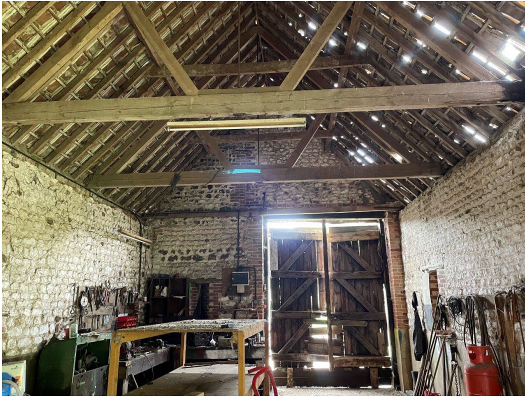
Photo 5: Interior – showing western gable
