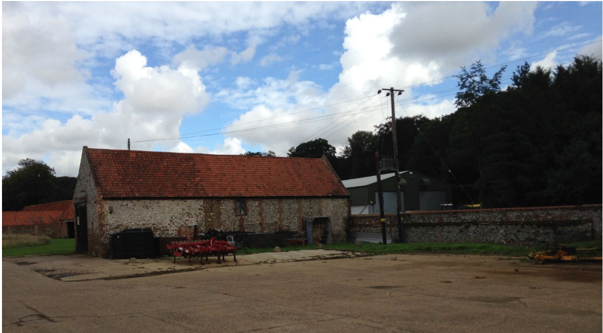
Photo 1: South elevation (facing farm yard)
