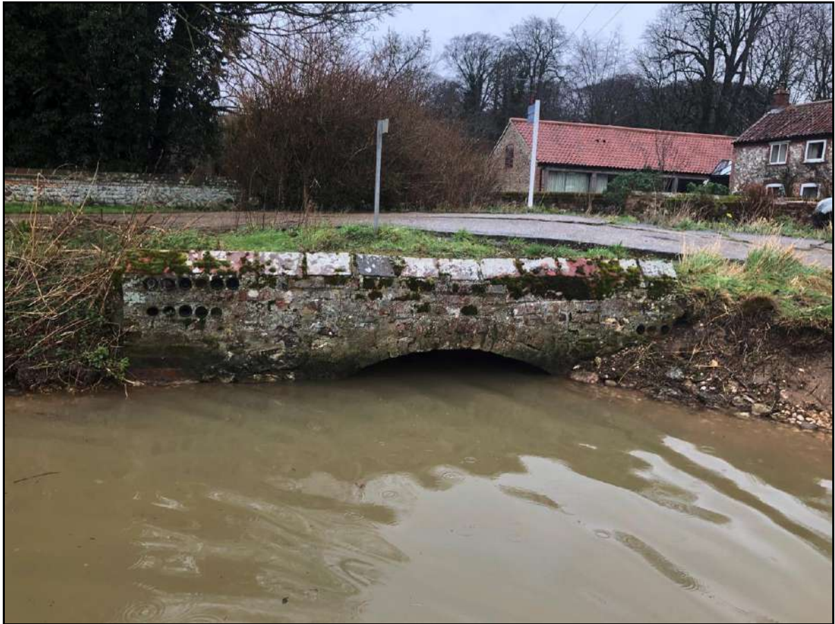
Figure 23: Bridge downstream of site
