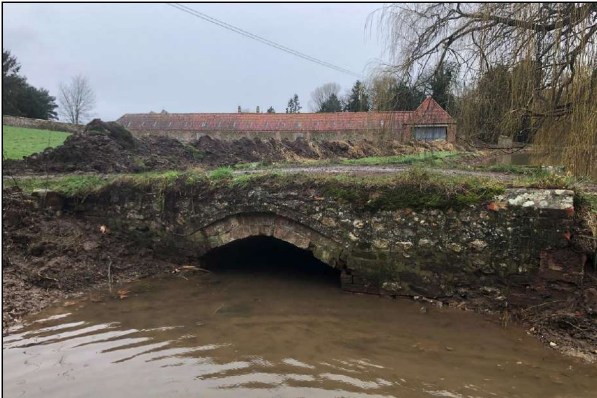
Figure 22: Bridge upstream of site with site in background
