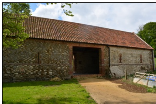
Figure 7 – Eastern view of Field Barn 2
