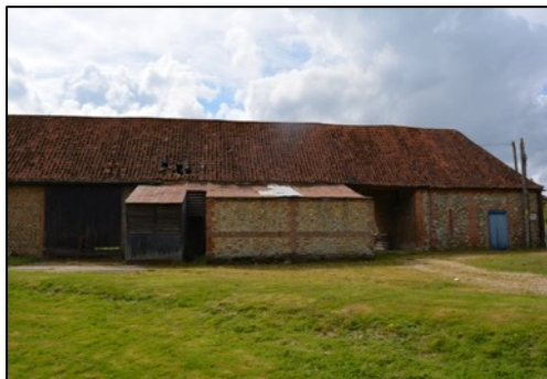
Figure 14 – Eastern view of Main Barn 4 Complex (sections A,B,C,D and K) and the mown lawn towards the east of barns
