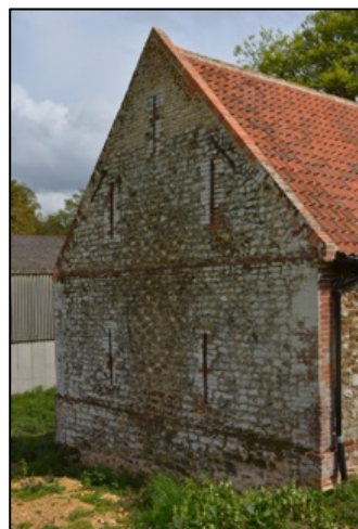
Figure 10 – Northern elevation of Field barn 2
