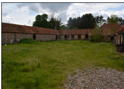
Figure 16 – North-west view of Main Barn 4 Complex (sections E, F and G) and the courtyard between them
