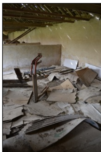
Figure 29 – Internal view of Main Barn 4 Complex (section J)
