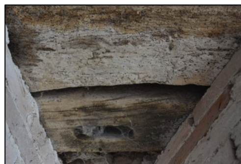
Figure 42 – Features between window lintels found on all windows
