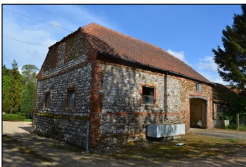
Figure 20 – North-western view of Barn 4 Complex (section I)
