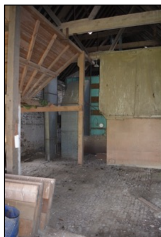
Figure 24 – Internal view of Barn 4 Complex (section C) including stored farming machinery
