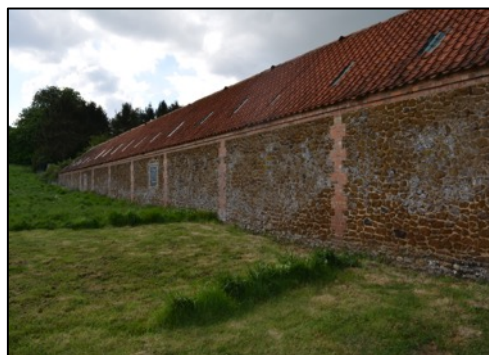
Figure 17 – Southern view of Main Barn 4 Complex (section E), showing a mix of cut and longer grass
