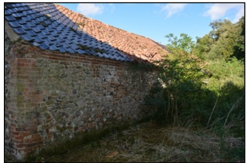
Figure 12 – Eastern view of Field Barn 3
