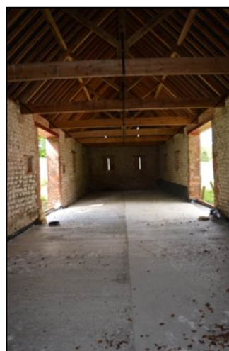
Figure 8 – Internal view of Field Barn 2 looking north
