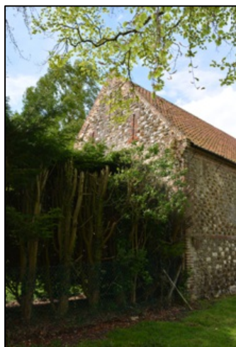
Figure 9 – Southern elevation of Field barn 2
