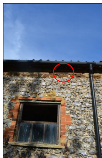
Figure 31 – Features where a single common pipistrelle was found within a mortar cavity on Main Barn 4 Complex (Section I)
