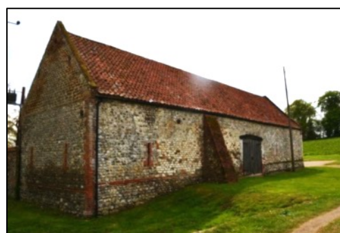
Figure 6 – Northern elevation of Field Barn 1
