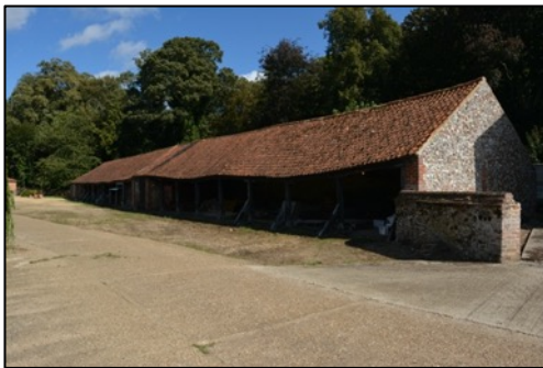
Figure 11 – Eastern view of Field Barn 3
