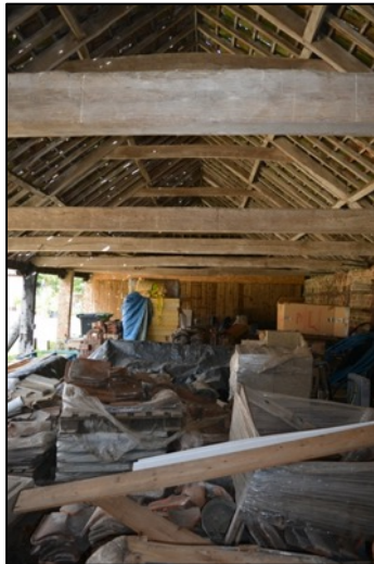
Figure 13 – Internal view of the northern barn of Field Barn 3
