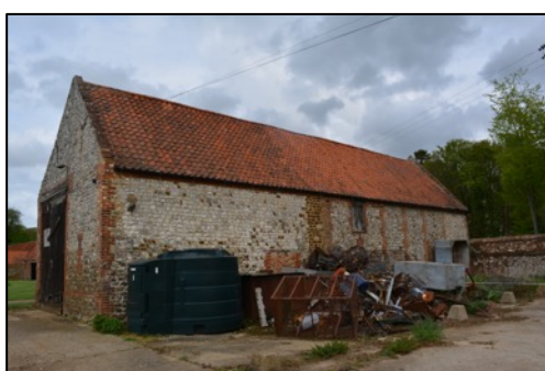
Figure 5 – Southern elevation of Field Barn 1
