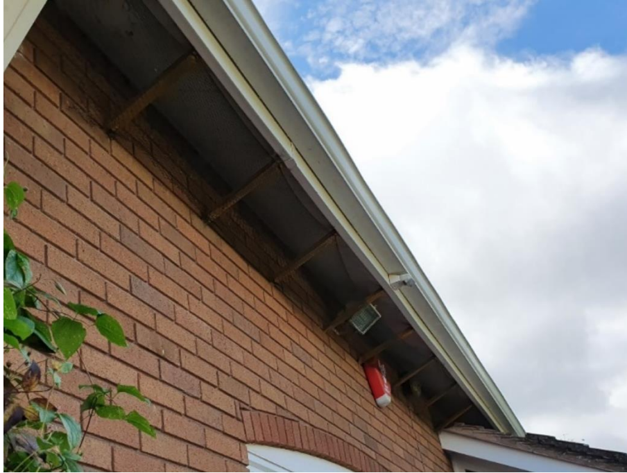
Figure 4.16. Netting under eaves
