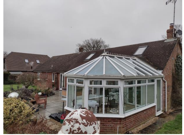
Figure 4: Southern elevation of the property
