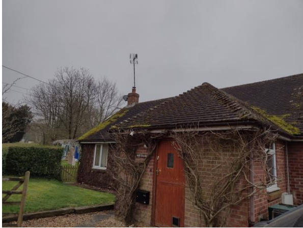
Figure 3: Northern elevation of the property
