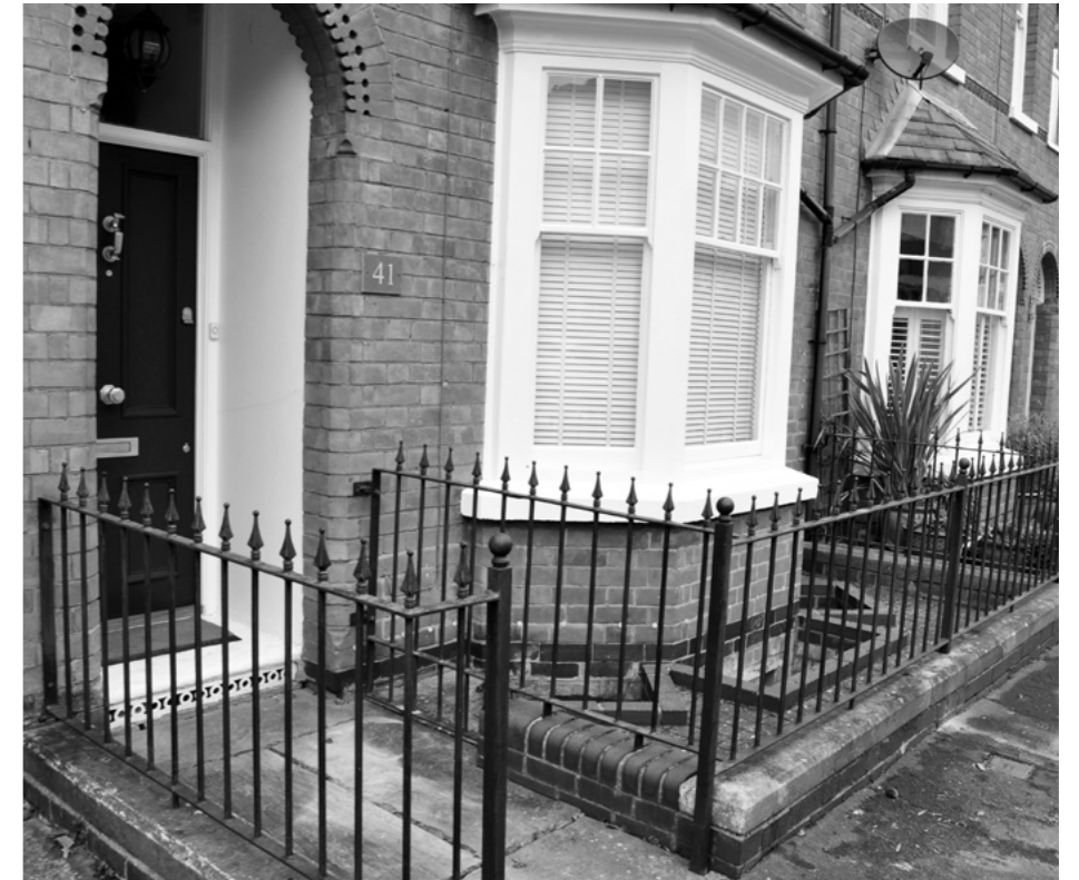
Figure 6/// Existing example of good principal elevation execution
