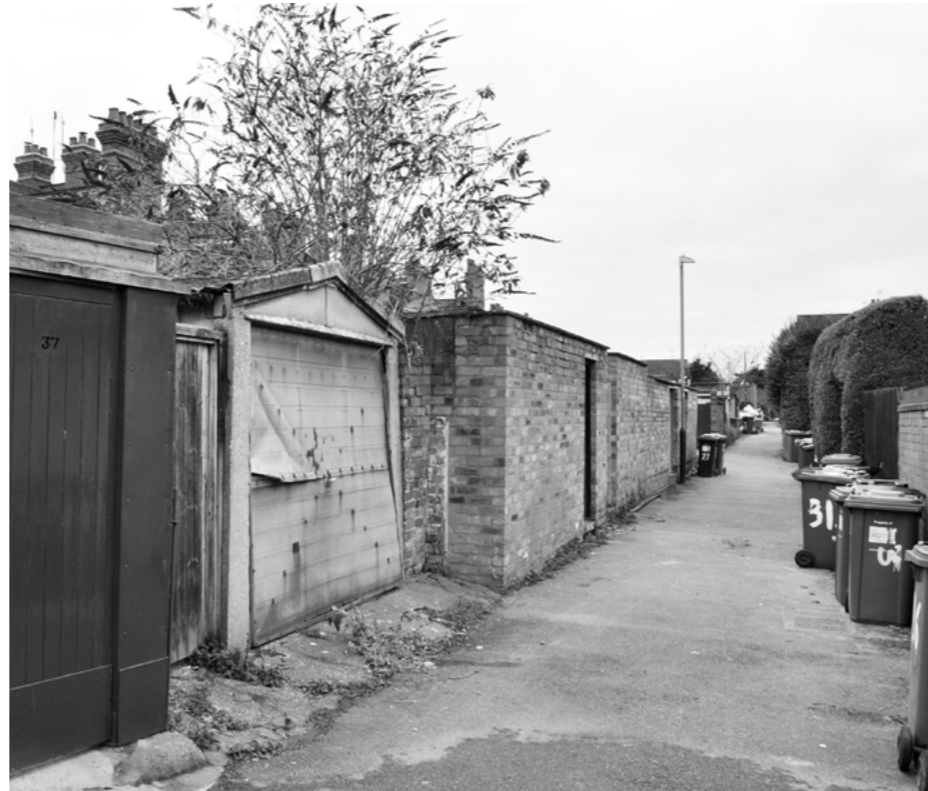
Figure 5/// Existing rear access linking Wathen and Campion Roads
