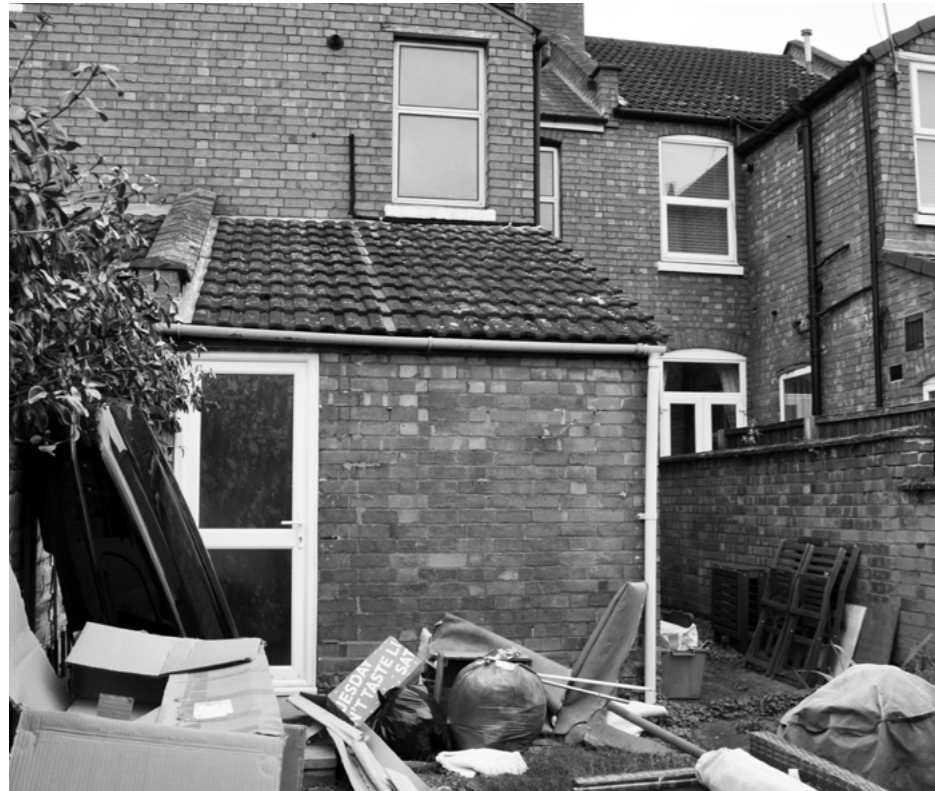
Figure 4/// Existing rear garden and current building condition
