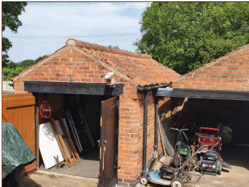
Photograph 3 - Southern aspect of buildings
