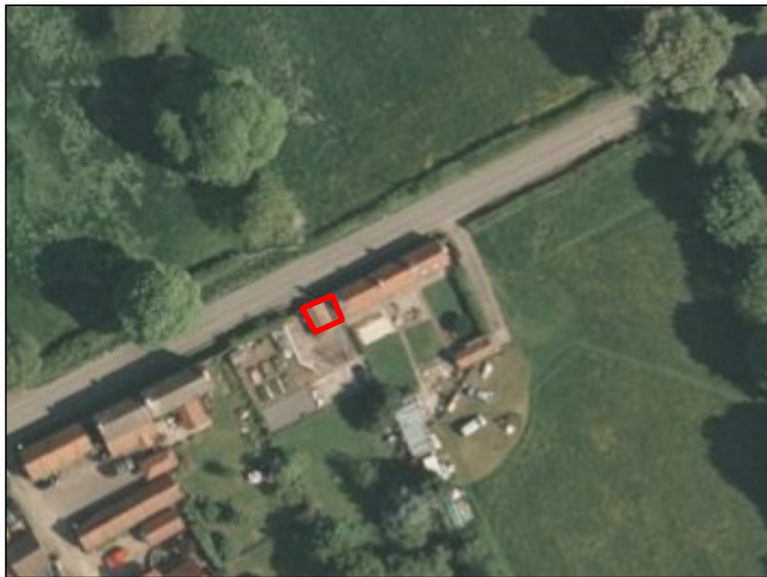
Plate 1 - Aerial view of site with buildings surveyed in red
