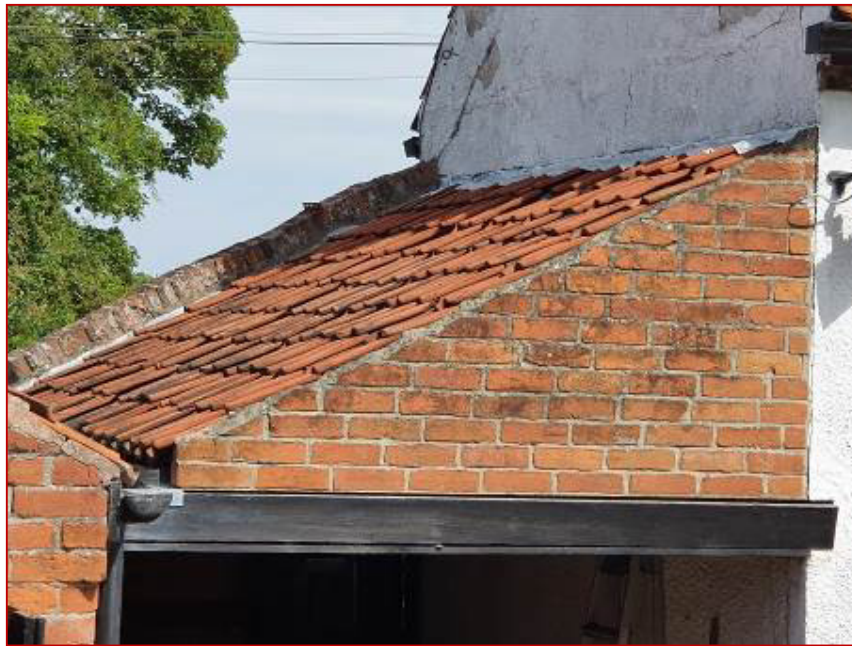
Photograph 2 - Roof of lean-to
