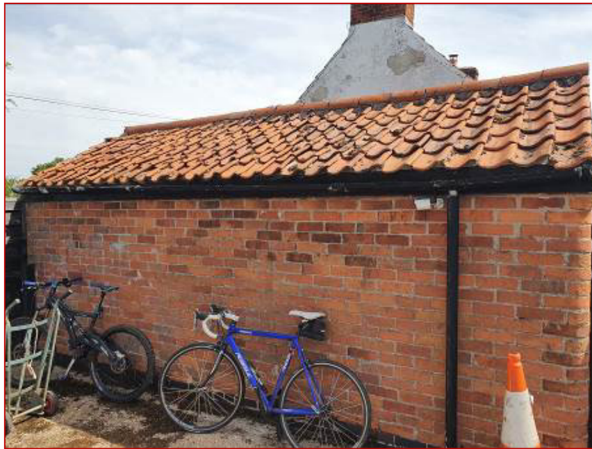
Photograph 4 - Western aspect of garage
