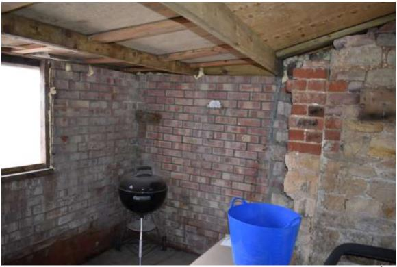
This shows the mix of stone and brick work construction, both modern, late 20<sup>th</sup> Century and of some earlier 20<sup>th</sup> Century. Note the poor quality construction, with straight joints in masonry and partially fixed wallplate straps.
