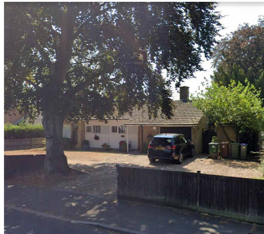
3. View of the front of the property from the street
