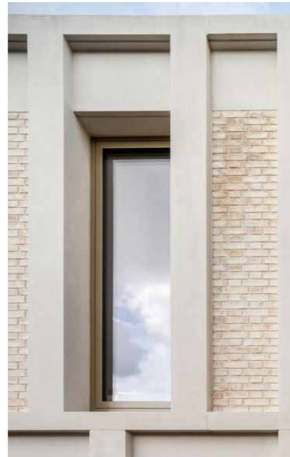
4. Pre-cast Concrete/Sandstone Cladding
