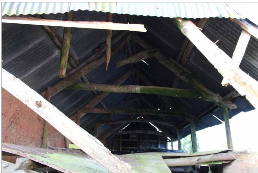
Plate 32: Roof structure of the linhay, looking west
