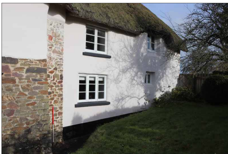
Plate 6: South elevation of the farmhouse, looking northeast (1m scale)
