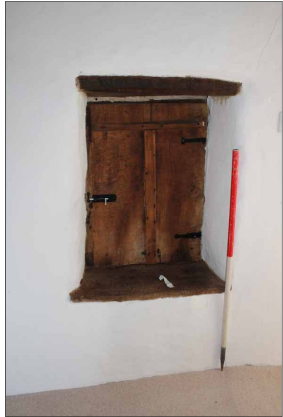
Plate 26: Window shutter in bedroom 4, looking south (1m scale)
