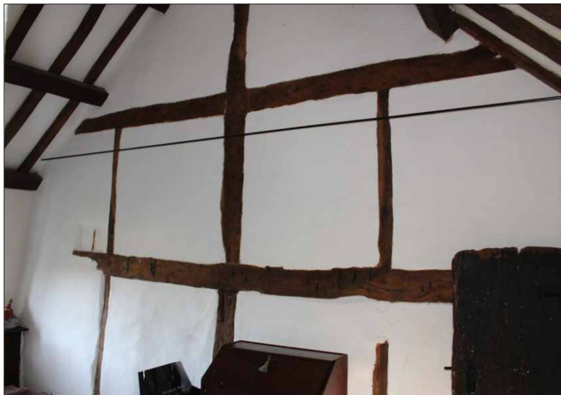
Plate 27: Timber-framed partition between bedrooms 3 and 4, looking west from within bedroom 3, looking northeast from within bedroom 4
