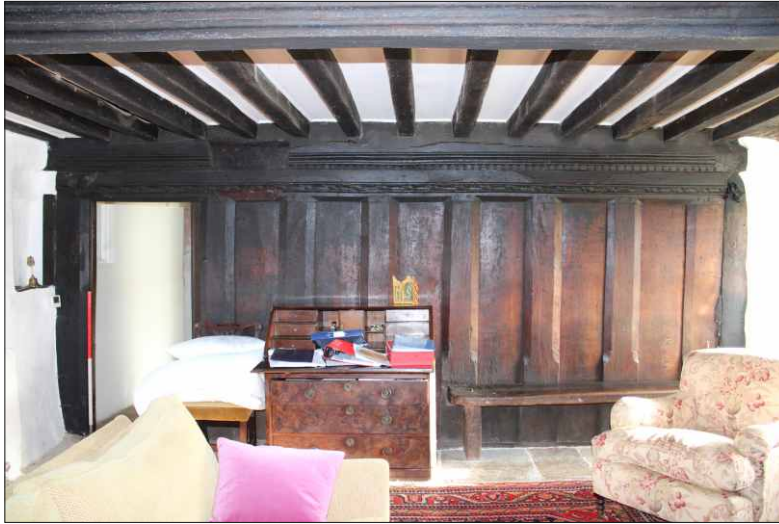
Plate 10: Screen in the hall, looking east (1m scale)
