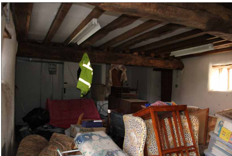
Plate 18: Shippon, looking southeast
