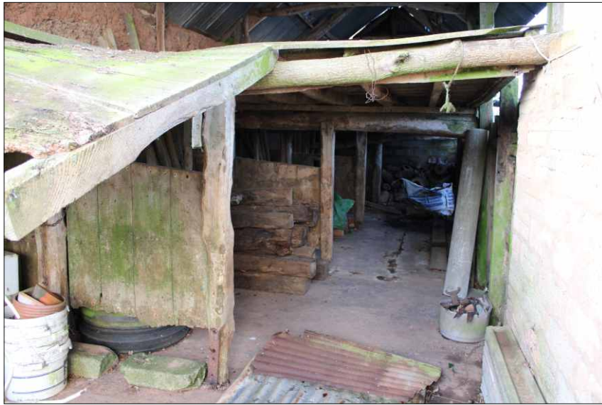
Plate 31: Ground floor of the linhay, looking southwest
