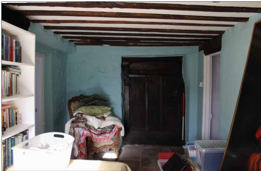
Plate 8: Cross passage, looking north (1m scale)
