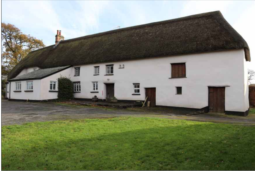
Plate 1: North elevation of the farmhouse, looking southeast (1m scale)
