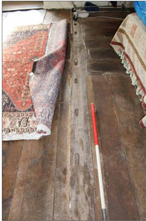
Plate 22: Line of former partition in bedroom 3, looking south (1m scale)
