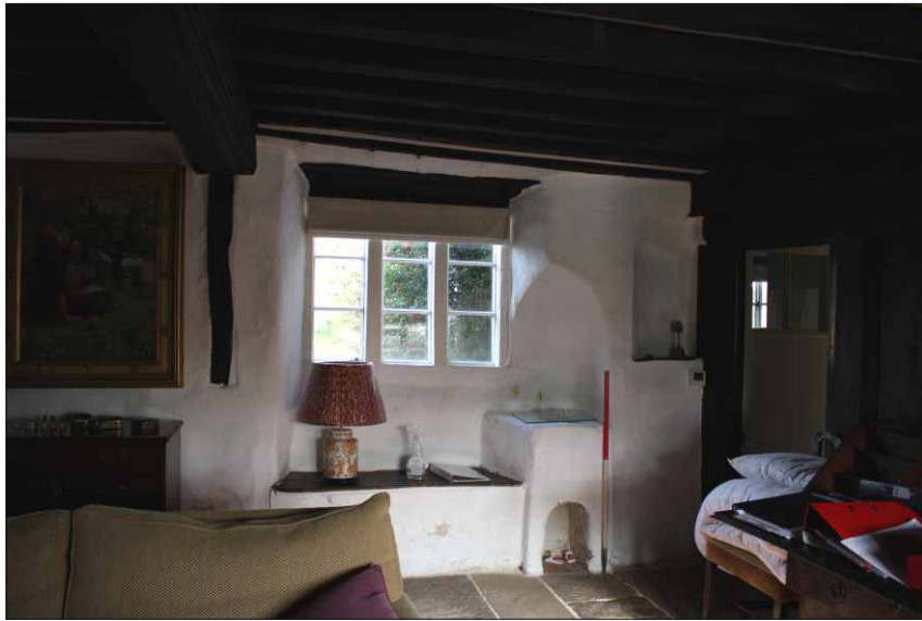
Plate 13: Northeast window and cream oven in the hall, looking north (1m scale)
