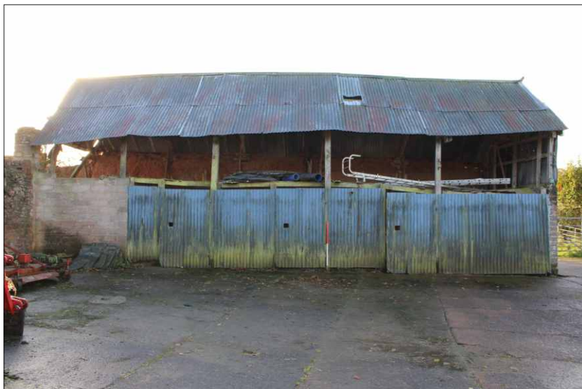
Plate 29: North elevation of the linhay, looking south (1m scale)
