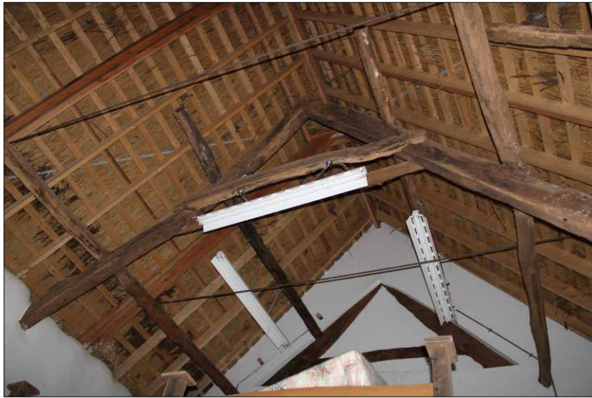
Plate 28: Roof structure of the shippon, looking northeast
