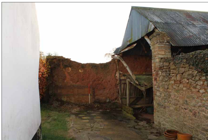
Plate 30: East end of the linhay showing how the south elevation continues beyond the current roof, looking south (1m scale)
