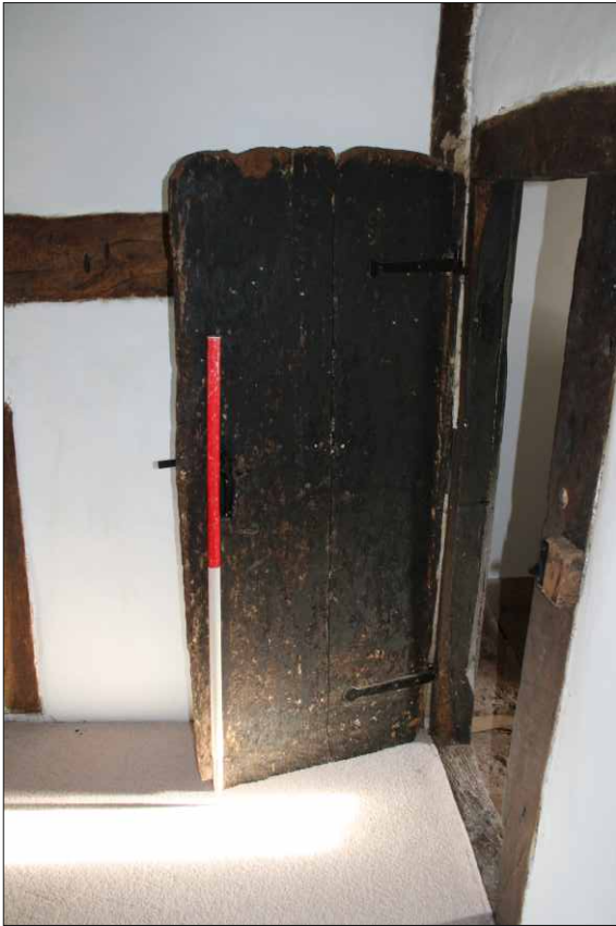
Plate 25: Door to bedroom 4, looking east (1m scale)
