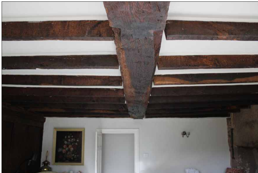
Plate 14: Bridging beam in living room, looking north
