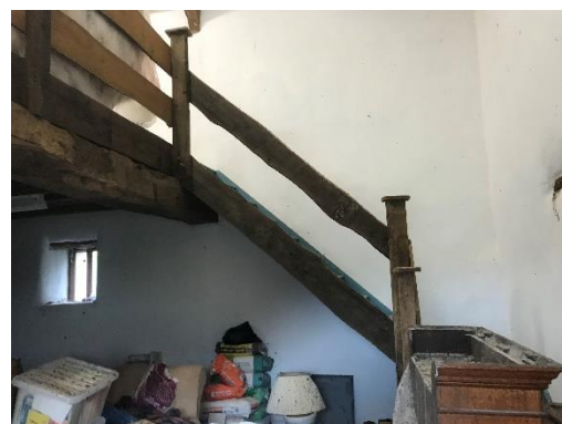
Shippon stair upto mezzanine
