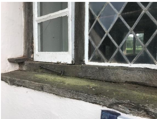
General repairs and decorations to historic frames and casements
