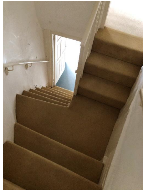
Half landing with steps to bed 1 and 2
