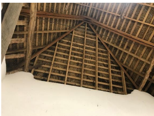
Shippon exposed roof structure
