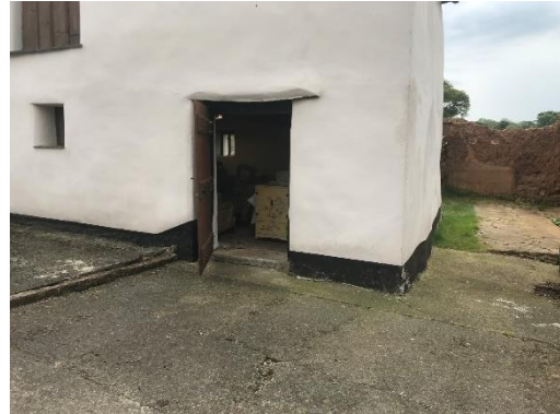
Modern boarded door into shippon to be replaced with 2-part stable doors on extended hinges. Full height fixed glazing unit to be fitted internally within reveal.
