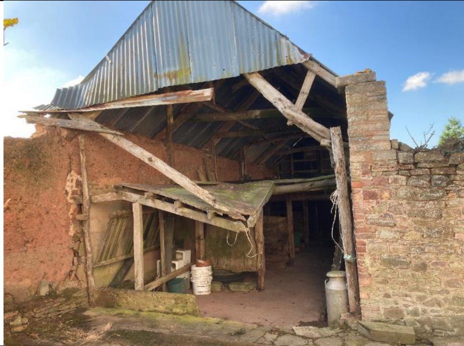
Photo 5: The linhay taken from the east.
