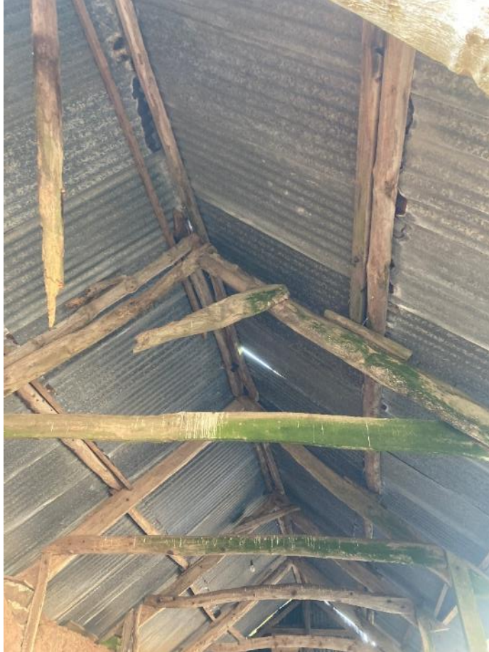
Photo 8: The internal linhay roof structure.
