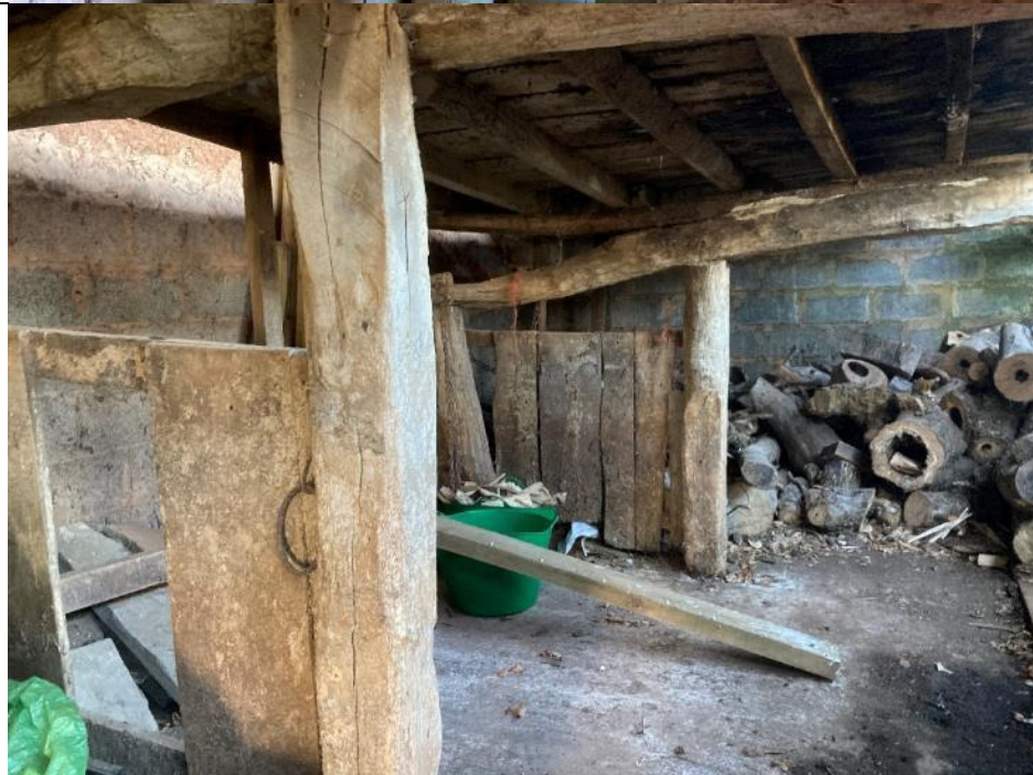
Photo 11: View of the lower level of the linhay, with wooden stalls.
