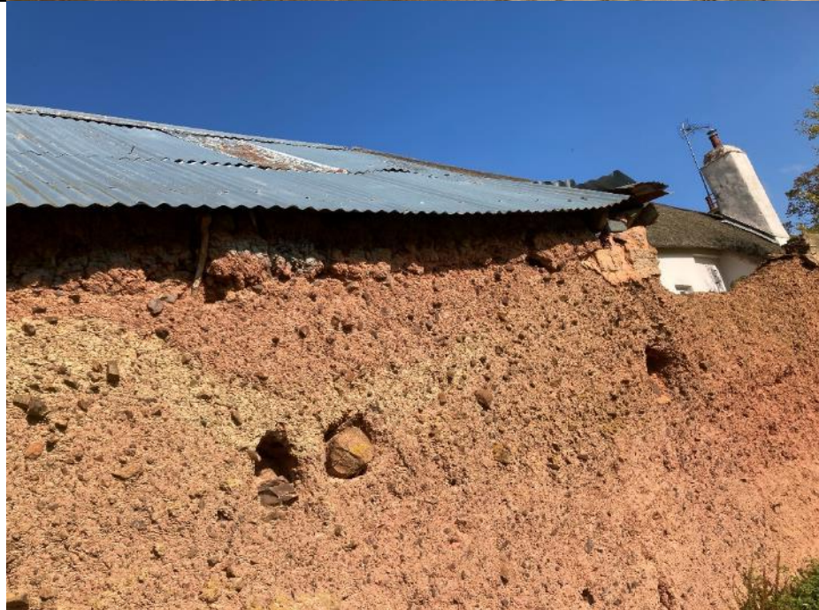
Photo 7: The cob linhay wall taken from the south.
