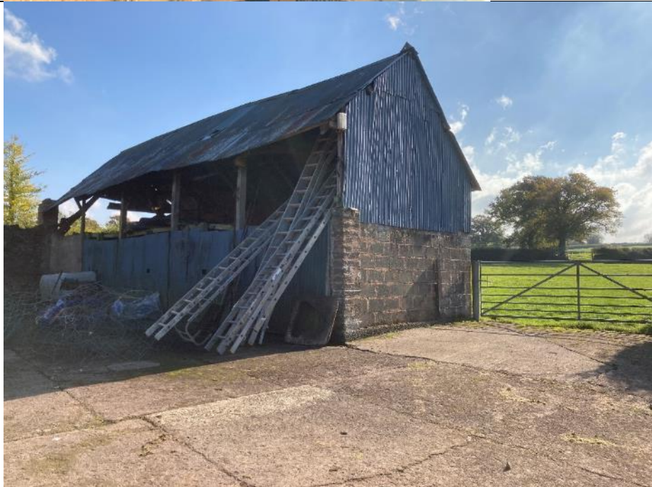
Photo 9: The linhay taken from the north-east.
