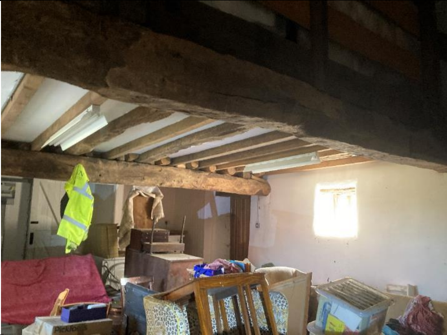
Photo 12: Internal view of the ground level of the stable block.
