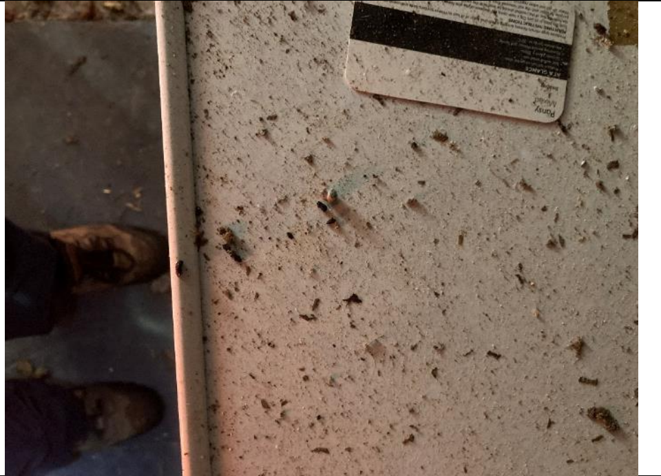
Photo 18: Further example of scattered bat droppings on stored items.
