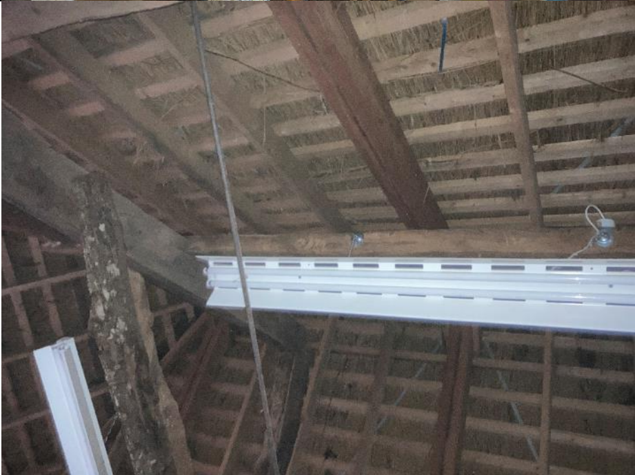
Photo 13: Internal view of the stable block roof structure.
