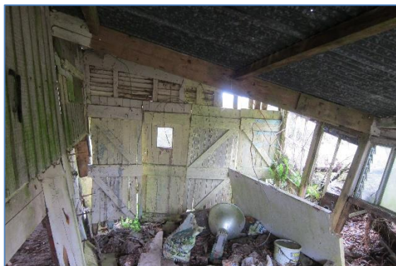
Single pitched roof attached to the west end
