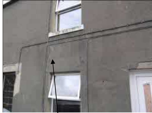
South Aspect Cracking
