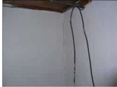
Bedroom South Wall Disengaging From Exterior Wall
