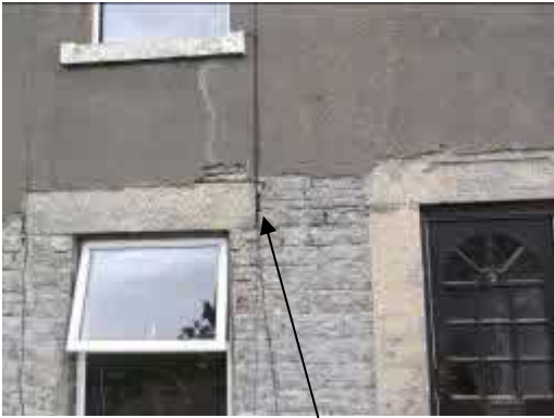
South Aspect Cracking
