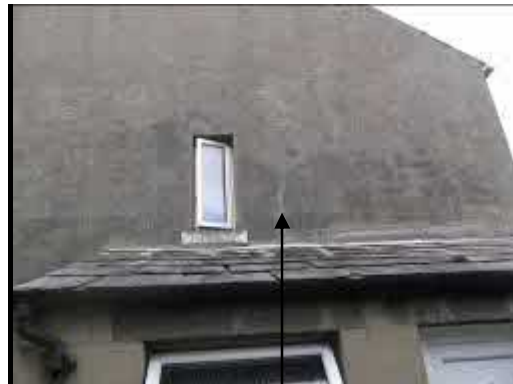
East Aspect Cracking
