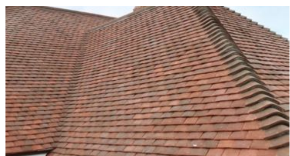
Proposed plain tile roofing
