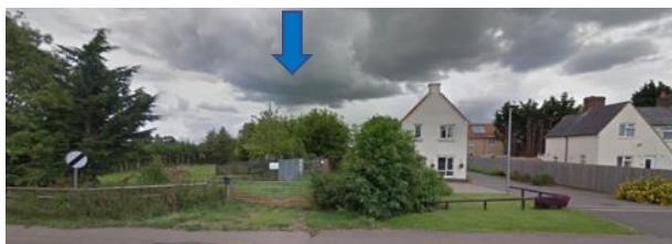
Fig 4. Plot 2. Location within streetscape. Site between 12 & 14 Bridge Road, Mepal, Cambridgeshire, CB6 2AR 12 Bridge Road, Mepal.
