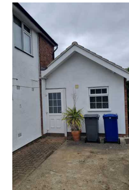
No. 35&37 School Road - Extensions
