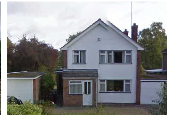
Neighbouring Building - No. 37 School Road
