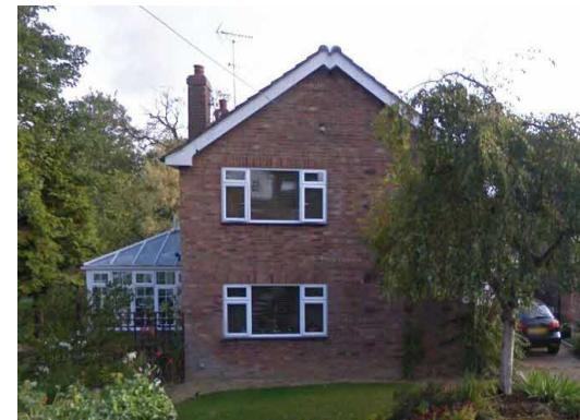
Neighbouring Building - No. 35 School Road
