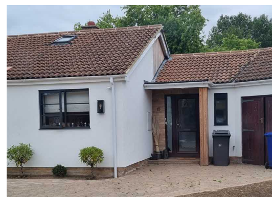
Neighbouring Building - No.15 School Road
