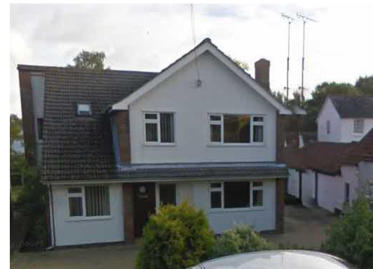
Neighbouring Building - No. 41 School Road
