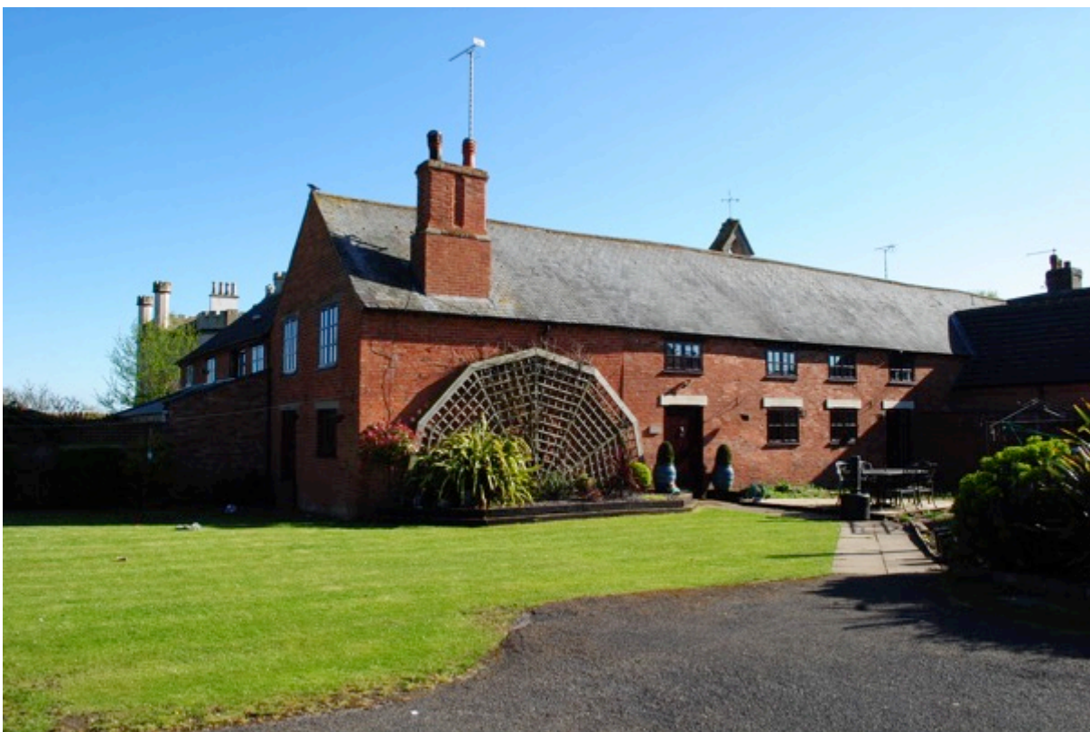
Plate 4: Study site: north and east elevations.
