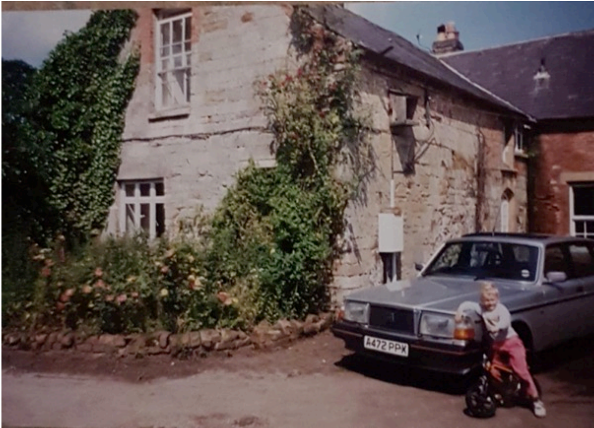
Plate 7: West wing (south), showing part of Chaworth Cottage (RHS, south elevation): Undated, but photograph likely taken around the 1970s. Source: client.
