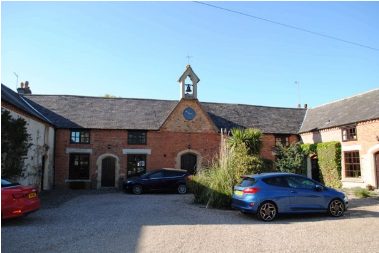
Plate 3: The study site, south elevation and main entrance (centre).
