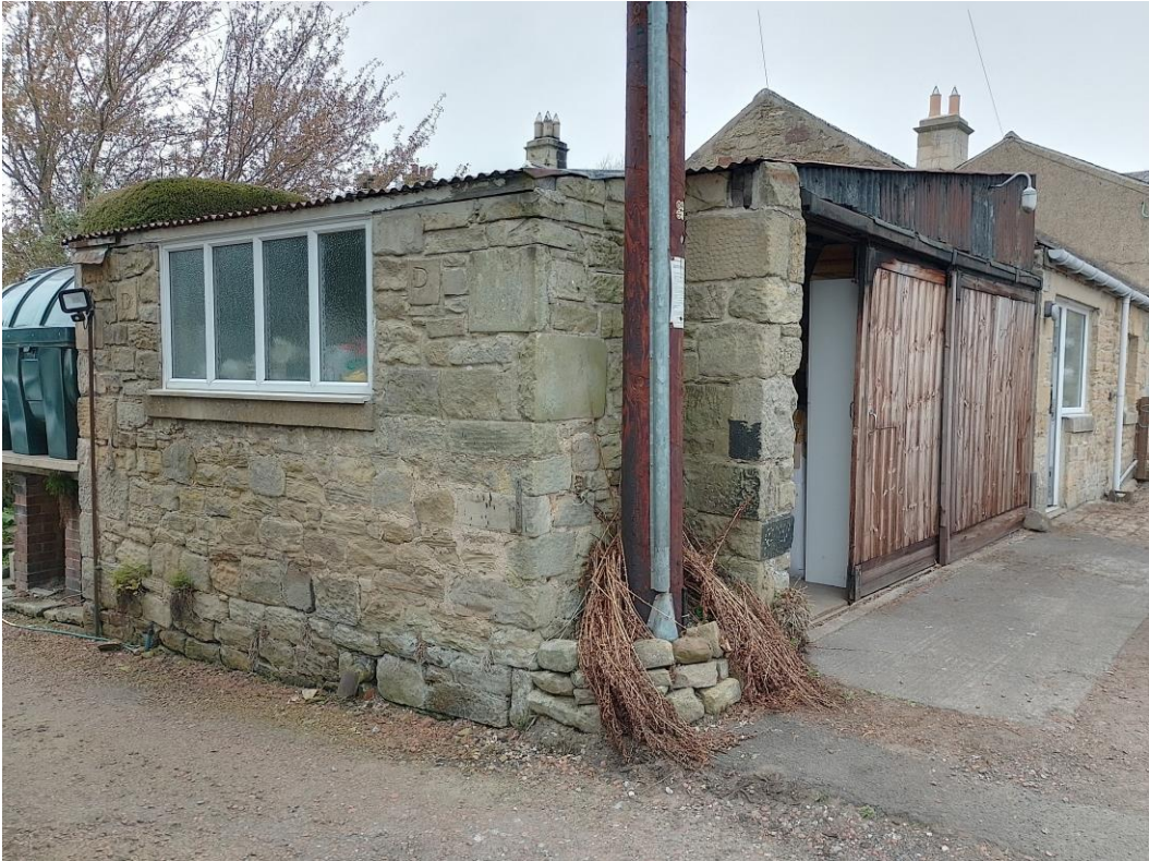
Elevation from Close House Drive
