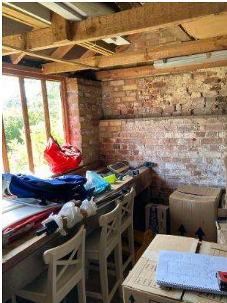
Internal masonry , note step
