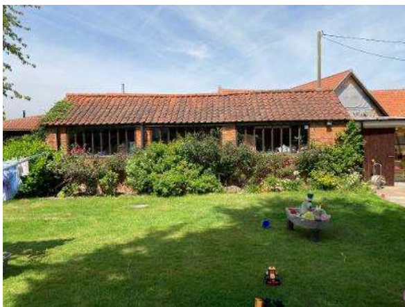
General view-front elevation
