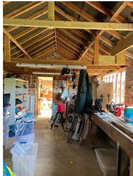
General view of roof and slab
