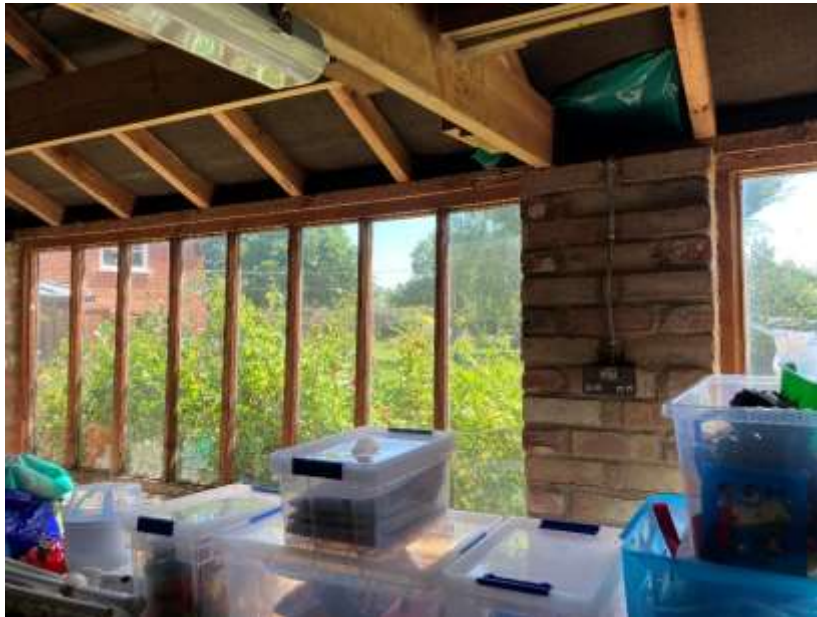
Window piers, note lintel
