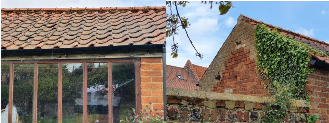
Fig 4. Pan tiles on east elevation (left) fig 5. South gable end (right)
