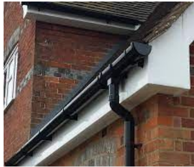
Black UPVC Guttering
