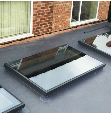
Flat roof lights
