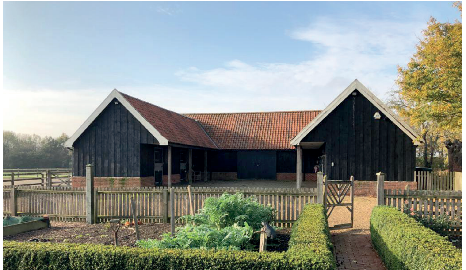
Top: Photograph of barn from kitchen garden (east)
