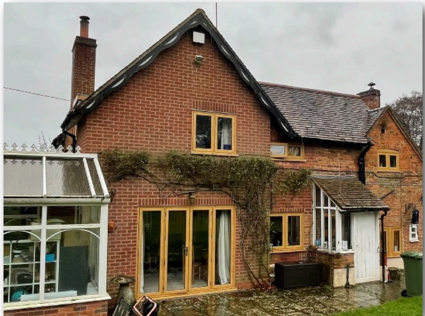
The photo above shows the first floor rear facing window within the existing extension, being clearly positioned away from the obvious central location.
