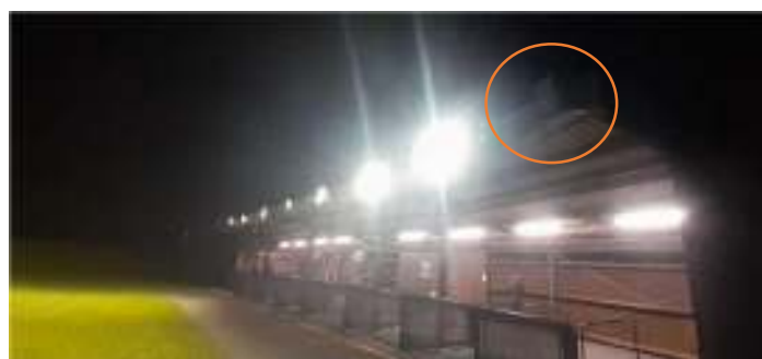
Figure 10 - Existing range lighting system failed light
