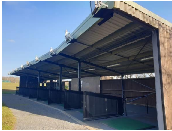
Photo 1 – Western elevation of B1.
