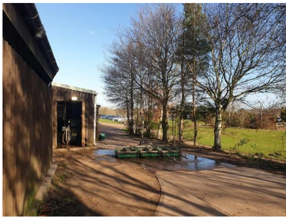
Photo 2 – Eastern elevation of B1, showing small extension.
