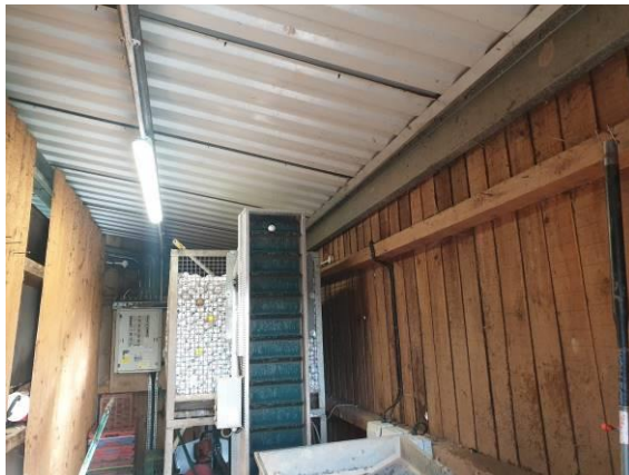
Photo 3 – Internal view of small extension.
