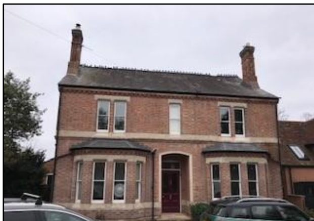
Plate 1: The front (eastern) elevation of the property. Photograph looking west.
