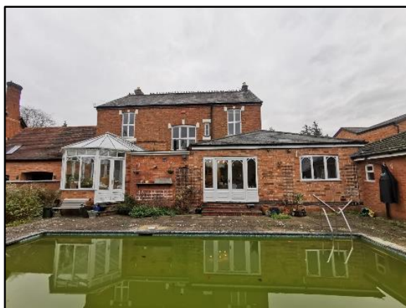
Plate 2: The rear (western) elevation of the property. Photograph looking east.
