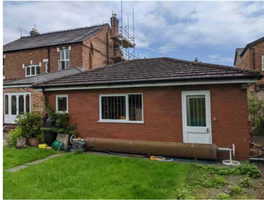
Existing Garage - Rear Elevation
