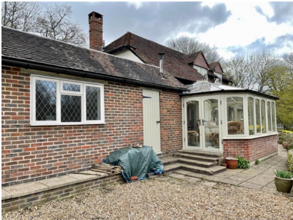
The west elevation of the earlier cottage, now much modified and later additions
