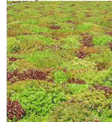
4.0 | Sedum roof - 40 m 2
