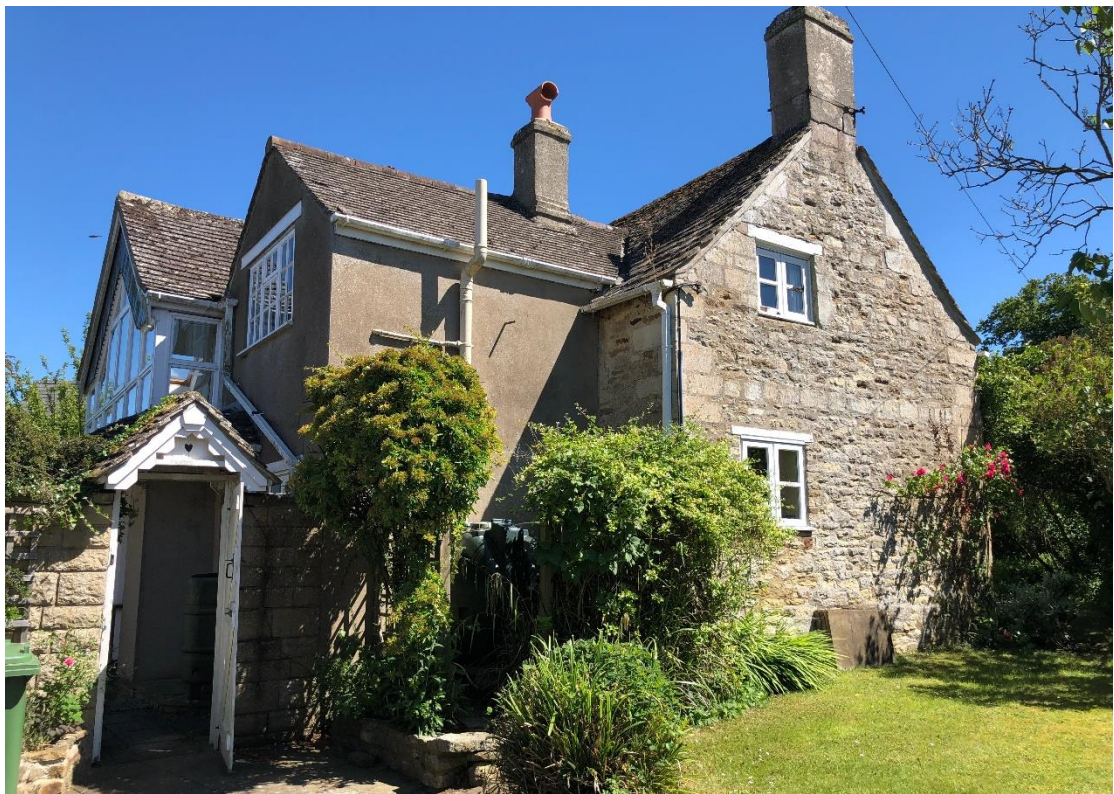
Above photo – existing side elevation.
