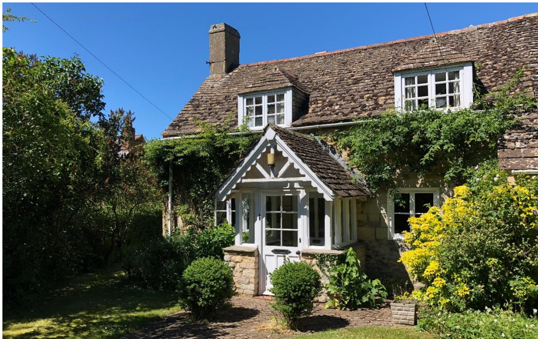
Above photo – portion of the existing front elevation.
