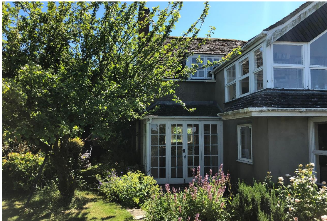
Above photos – portions of existing rear elevation.
