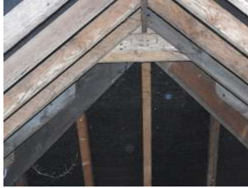
Fig. 28 Cobwebbed ridge and plumb cut of the extended hip to the north
