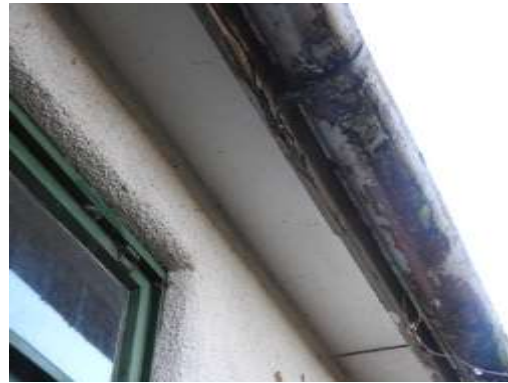
Figs. 20 & 21 Tightly fitting boxed soffits
