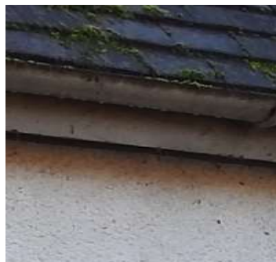
Fig. 22 Sealed eaves of the garage
