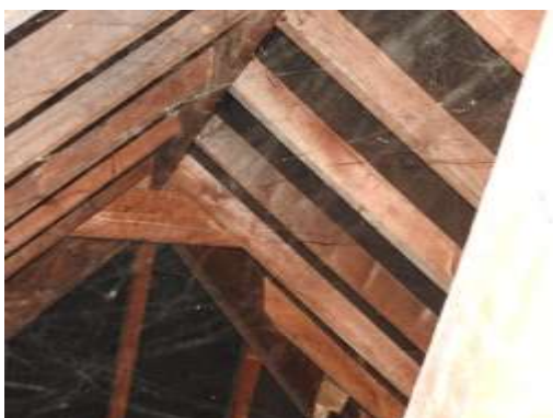
Figs. 26 & 27 Cobwebbed ridge and plumb cuts of the extended hips
