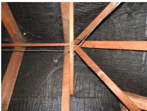
Figs. 24 & 25 Cobwebbed plumb cuts of the main roof
