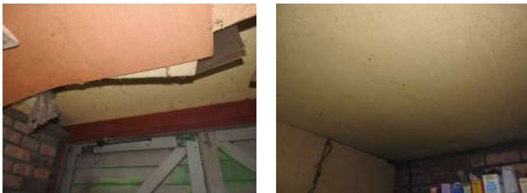
Figs. 28 & 29 Board lined underside of the flat roof
