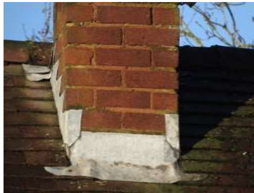
Fig. 19 Tightly moulded lead flashing around the base of the chimney
