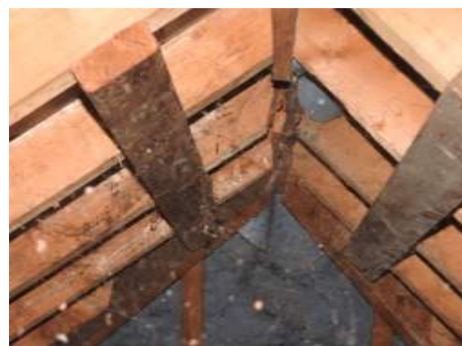
Figs. 26 & 27 Cobwebbed ridge and plumb cuts of the extended hips
