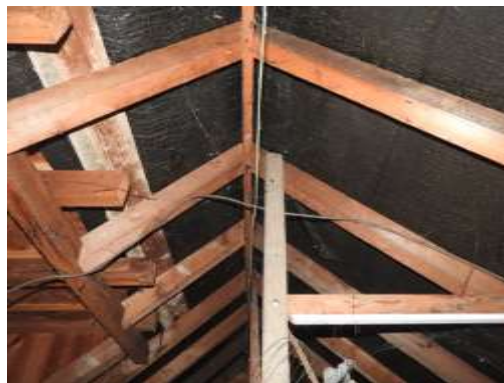
Fig. 23 Cobwebbed ridge of the main roof
