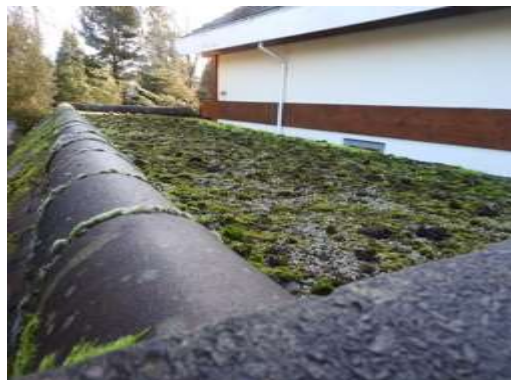
Figs. 17 & 18 Ridge and roof tiles of the garage (L) and the moss covered flat roof (R)
