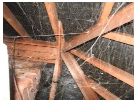
Figs. 24 & 25 Cobwebbed plumb cuts of the main roof
